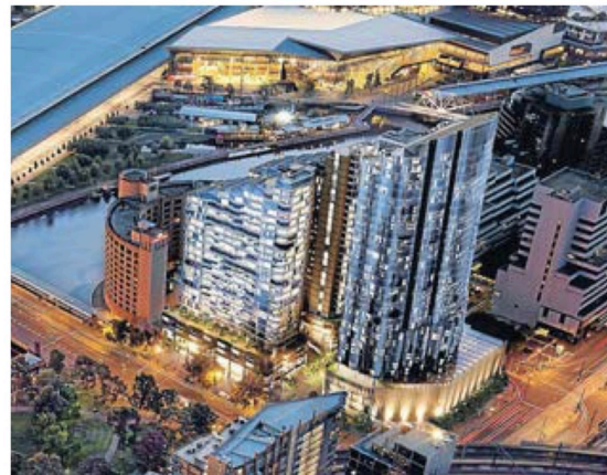
The Century Group apartment and hotel complex on Melbourne's Spencer Street.
