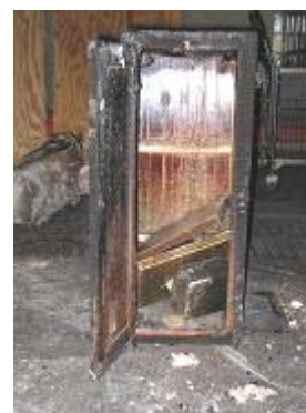
Cabinet (post fire)
