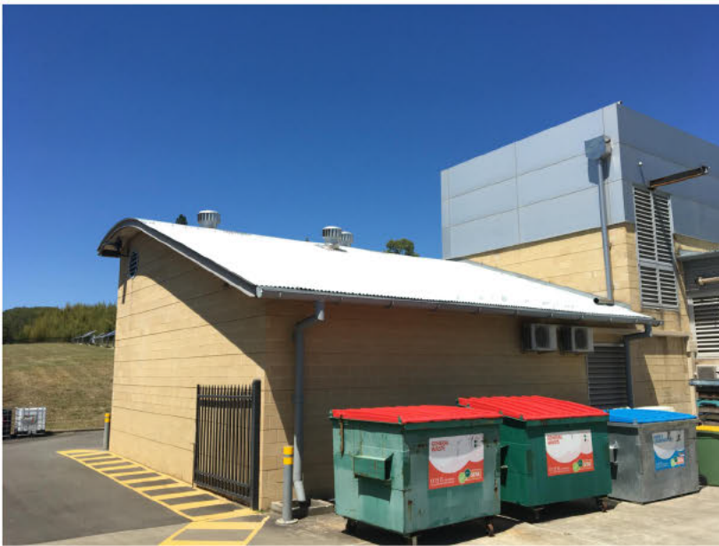
PHOTO OF EXISTING BATTERY ROOM & SURROUNDS PROPOSED REFURBISHMENT FOR SMOG CHAMBER
