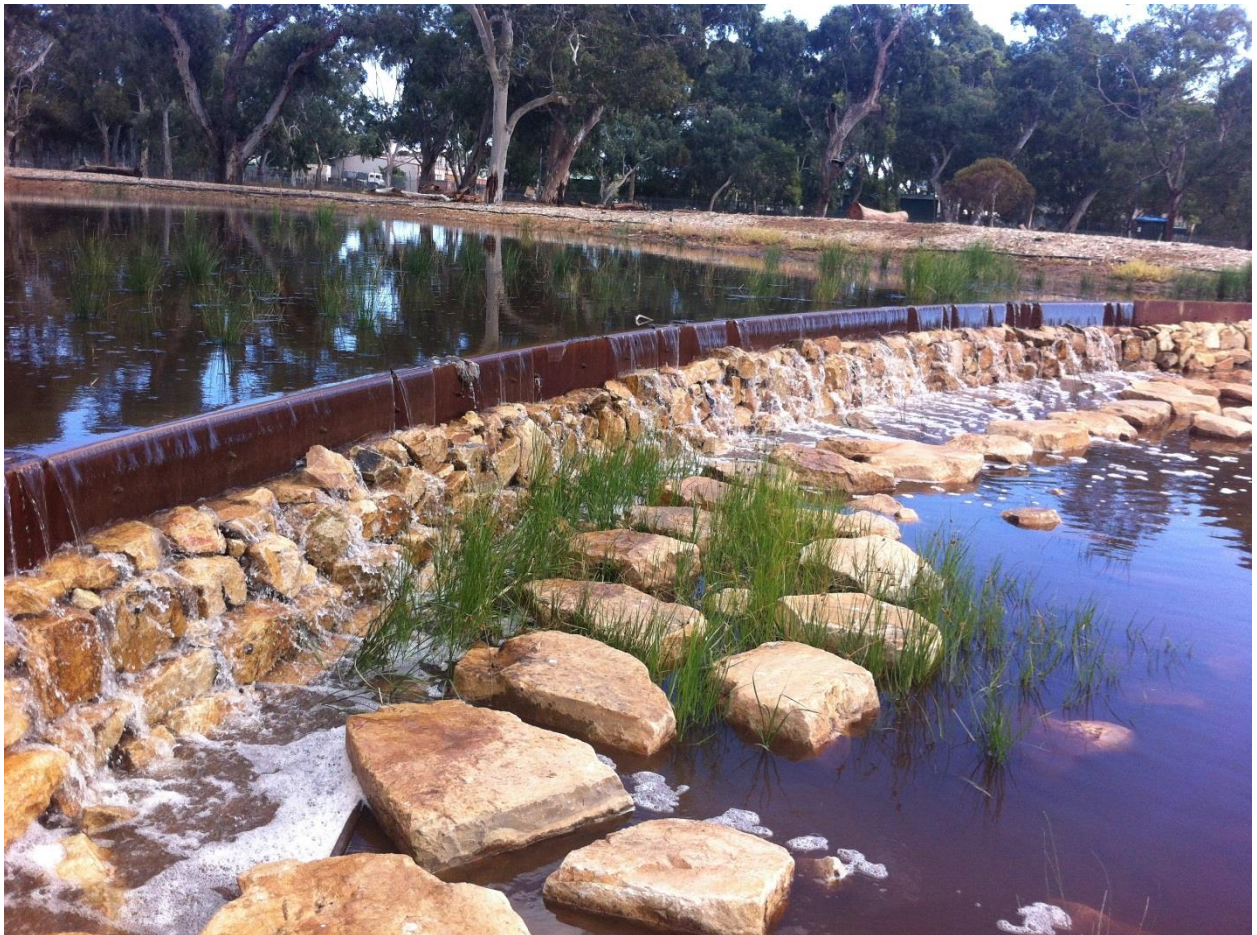
Oaklands Park stormwater harvesting wetland in SA – example of retrofit stormwater system with multiple benefits
