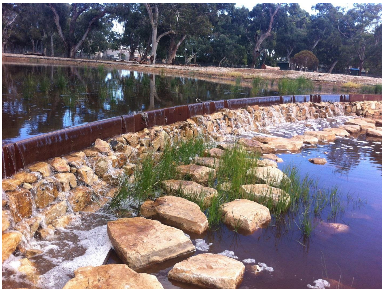
Oaklands Park stormwater harvesting wetland in SA – example of retrofit stormwater system with multiple benefits
