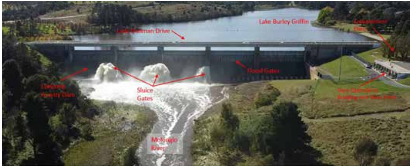
Figure 2.3 General arrangement of Dam
