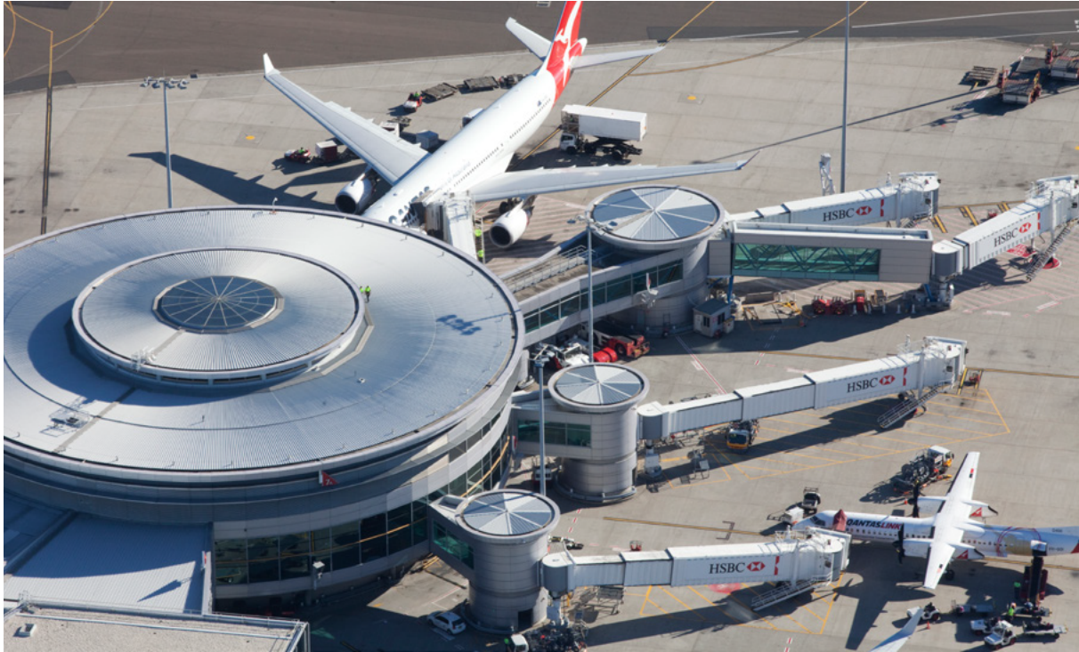
Sydney Airport, New South Wales.
