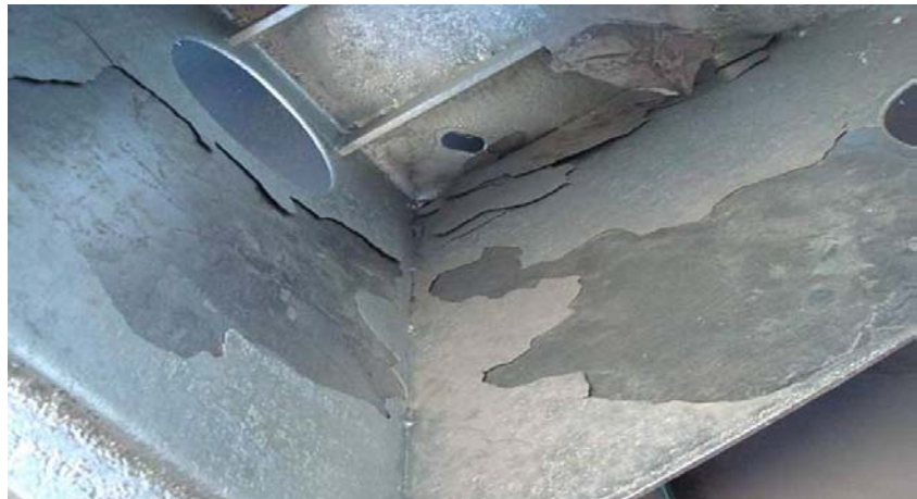
Photo 2 Poor galvanizing due to steel chemistry
