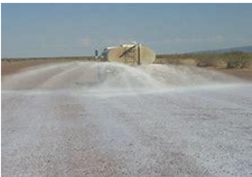
Construction site dust control
