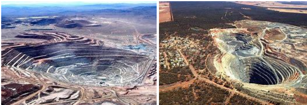
Open cut lithium mines
