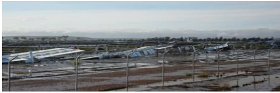
Storm damage to a PV solar IEGW
