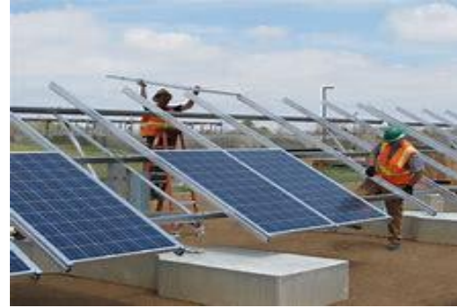
Crew of two install cross-members and panels
