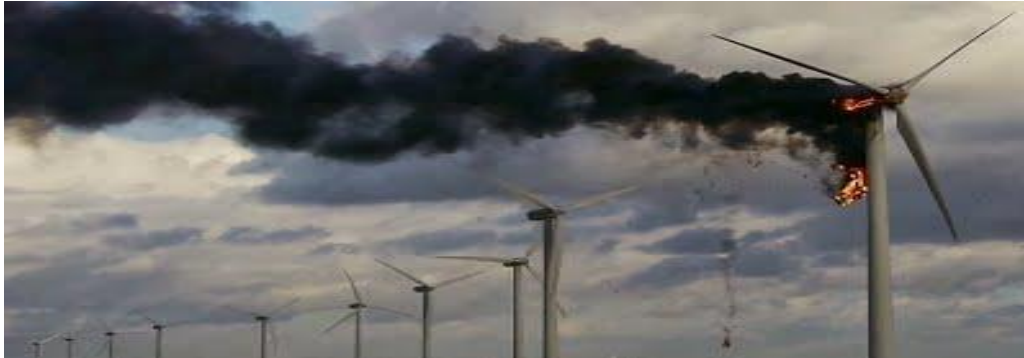
Wind turbine on fire
