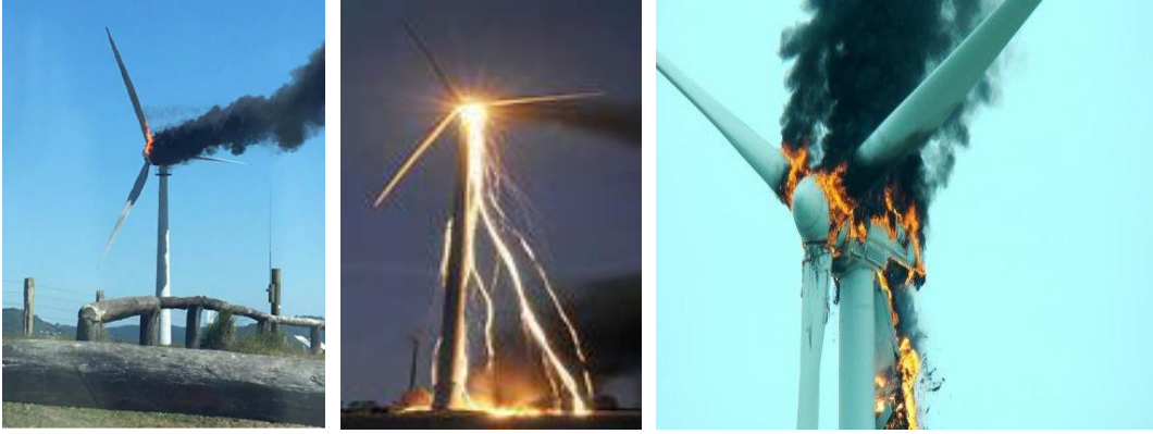
Burning wind turbines can easily result in starting devastating bushfires or grass fires in rural areas
