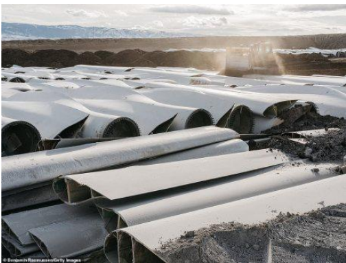
Disposing of cut up wind turbine blades
