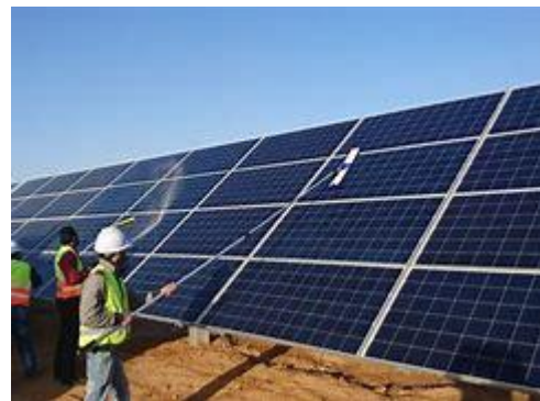
Cleaning PV solar panels
