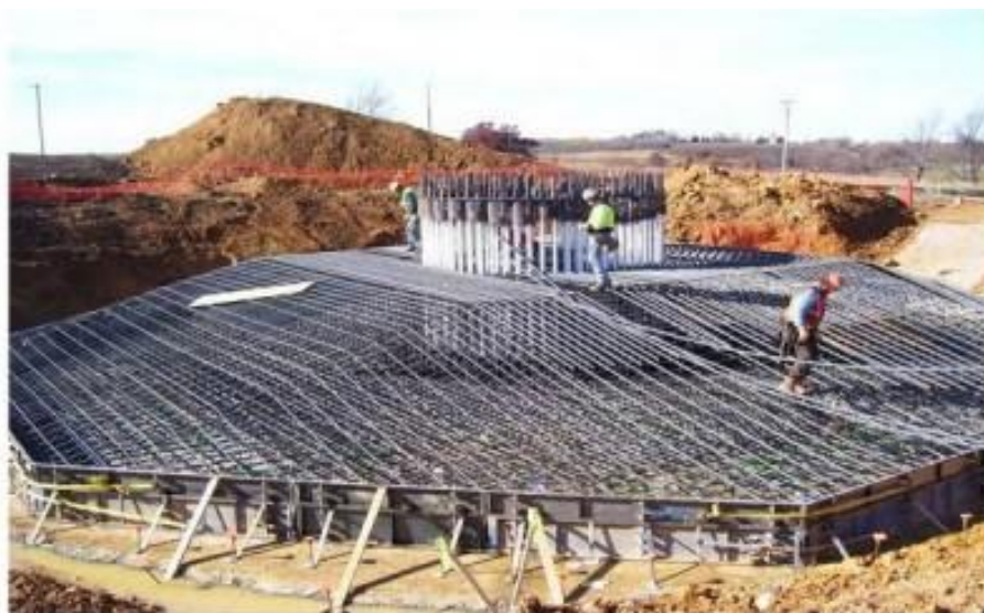
A single wind turbine concrete base under construction
