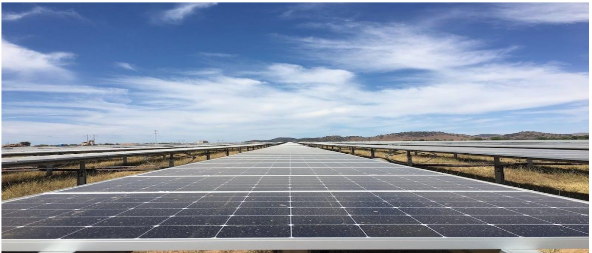
Beryl PV Solar Industrial Electricity Generating Works, Central West NSW
