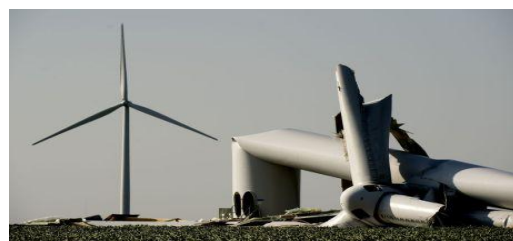
Wind turbine collapse
