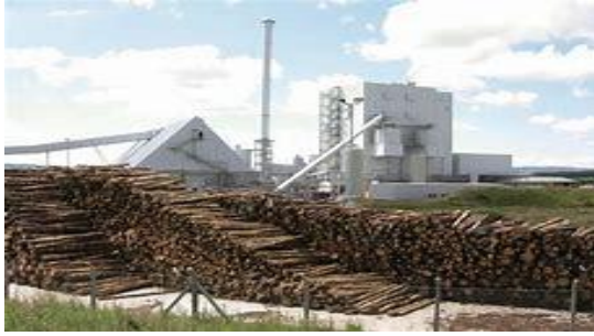
Biomass power plant
