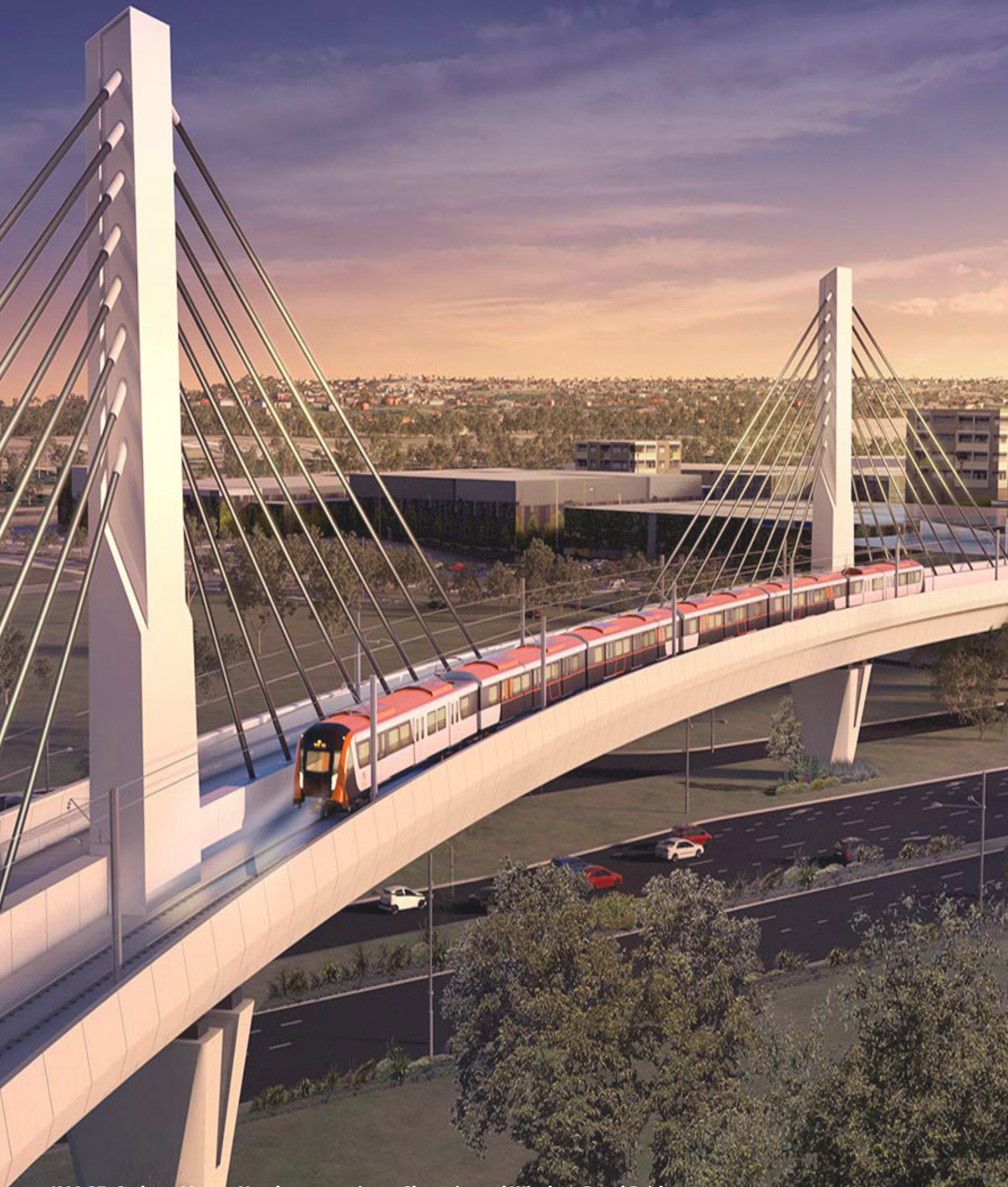
IMAGE: Sydney Metro, Northwest project - Skytrain and Windsor Road Bridge. The $340 million skytrain will include a 4km stretch of raised rail between Bella Vista and Rouse Hill. The Windsor Road Bridge will be 270 metres long, up to 45 metres high and will be supported by 32 steel cables.
