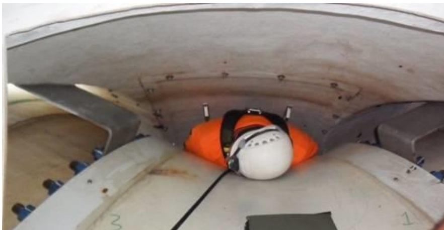
Figure 10- Maintenance worker crawling over the top of the Hub to access the inside of the Hub
