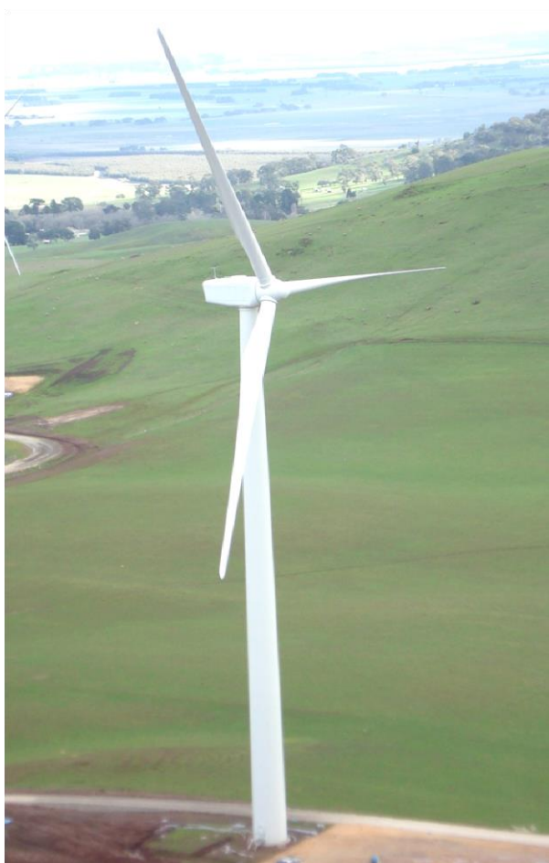
Figure 1-An 80 meter high wind turbine
