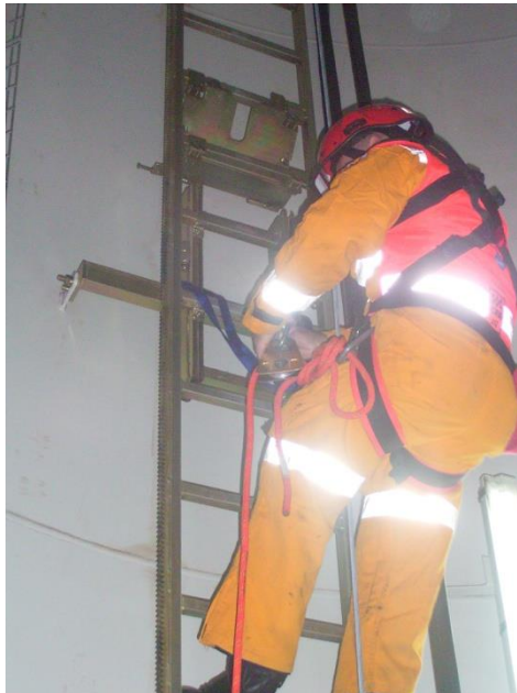
Figure 3- Ladder fixed to side of tower. Climbers back towards the inside of tower
