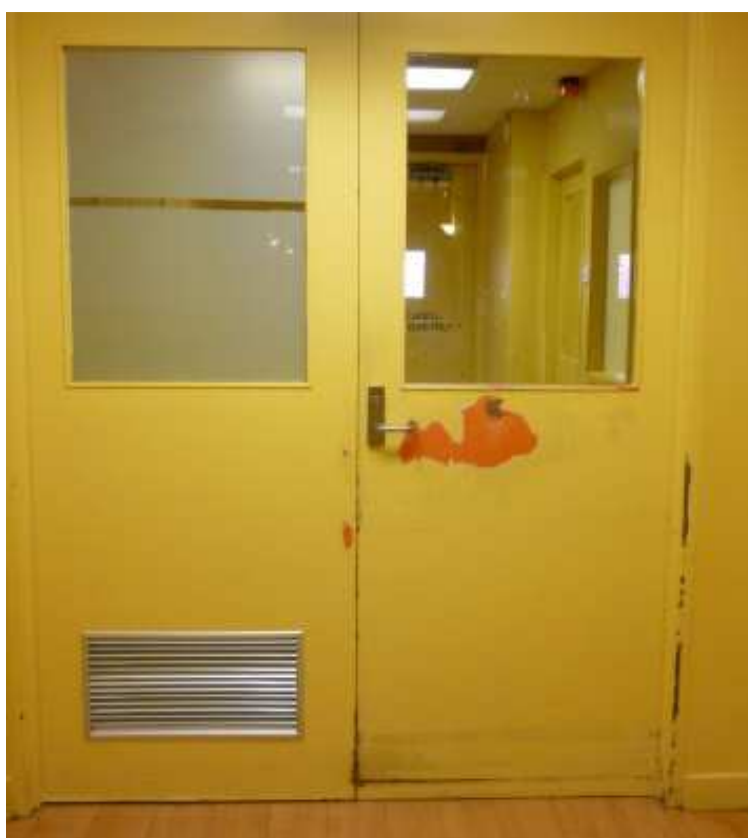
Image 7: Door, door jambs and walls
