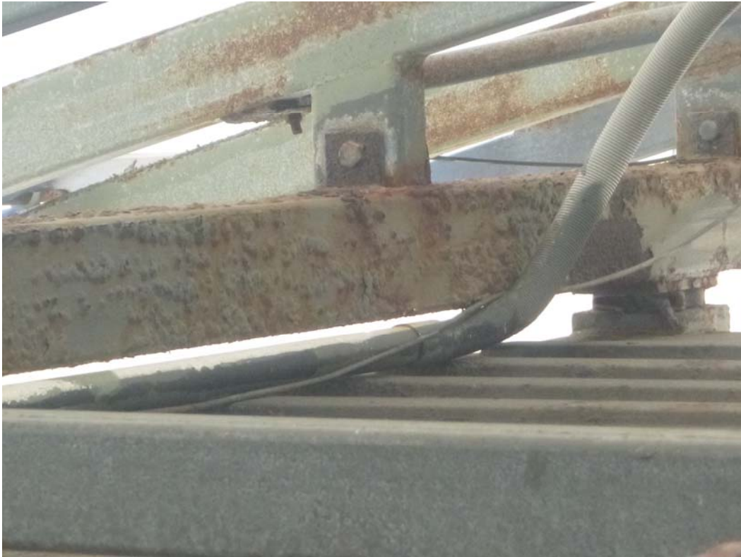
Figure 3: Examples of corrosion issues and damage at the existing temporary ARFF facility at Hamilton Island
