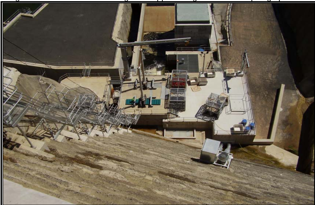
Image taken from above the upstream fishway indicating the steep angle of attack for spilling and stepped design , with cable arrangement for hauling upstream fish cage over dam wall ,shown in left of image .
