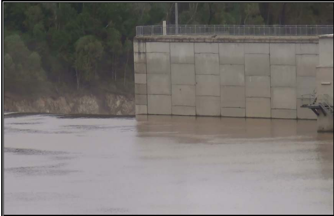
Image C taken on Feb 30 th 2013 indicating flood level stain marking within 1 meter of overtopping the wall . Concrete blocks are 2.00 M in Height. BOM website indicates a peak level above the spillway of 8 M,
