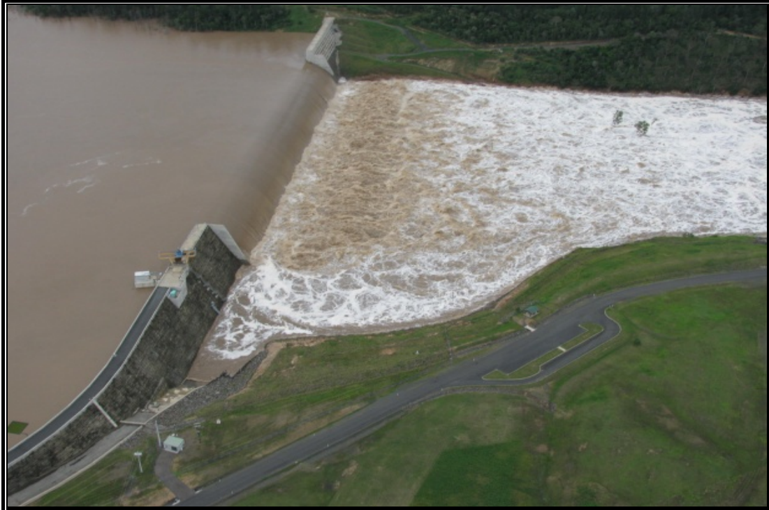
Image A of flood level December 30 th 2010 indicating control system inundation, image courtesy of Hubert Chanson .
