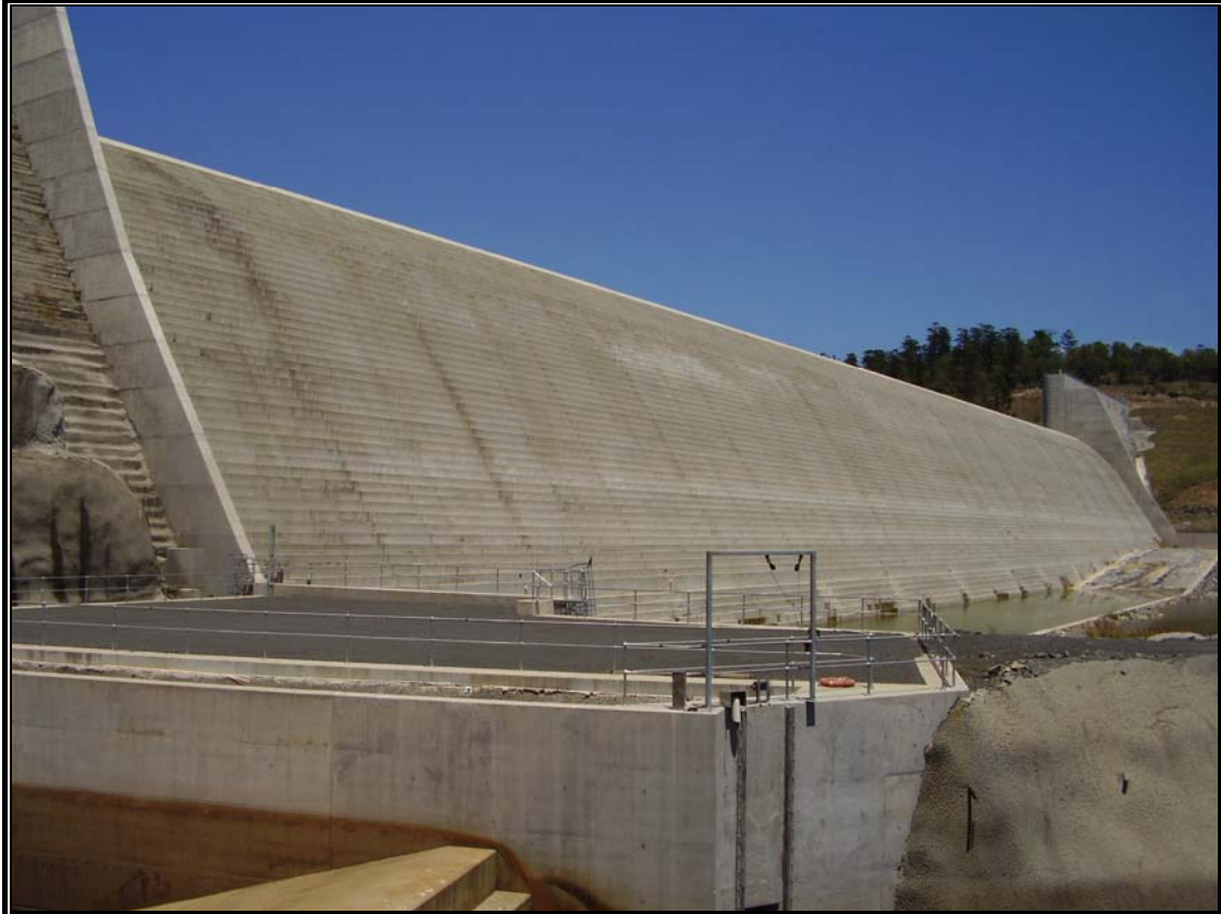
Image taken at the dam indicating the stepped design and shallow plunge pool .
