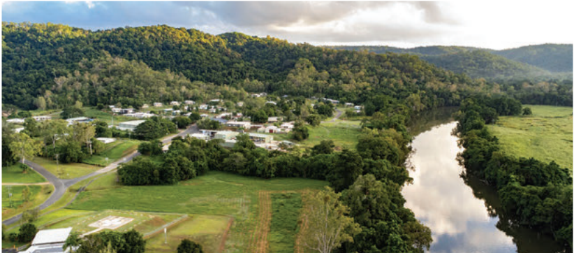
Aerial view of Wujal Wujal
