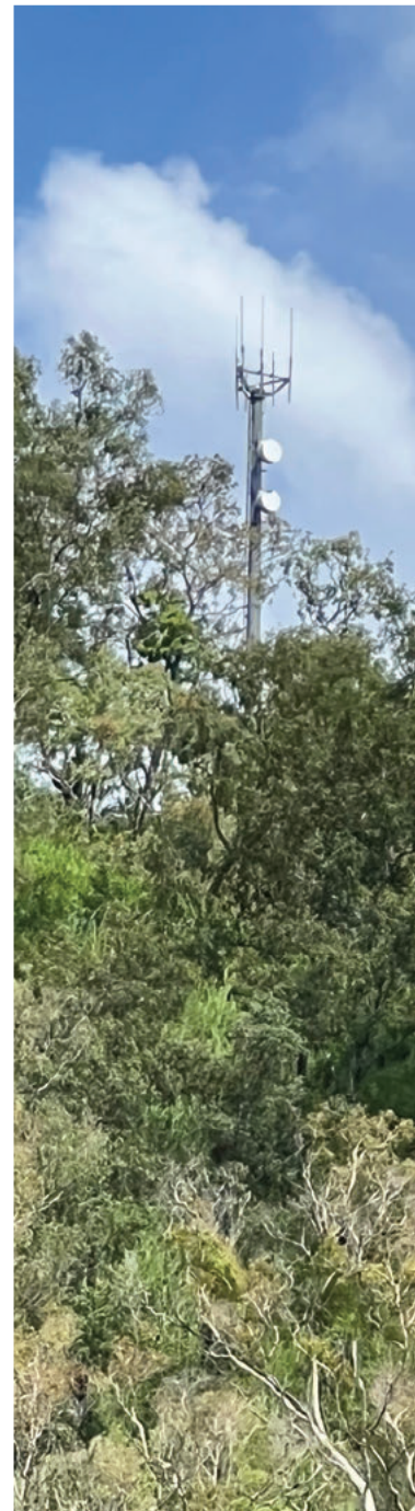
Mobile tower in Wujal Wujal, QLD
