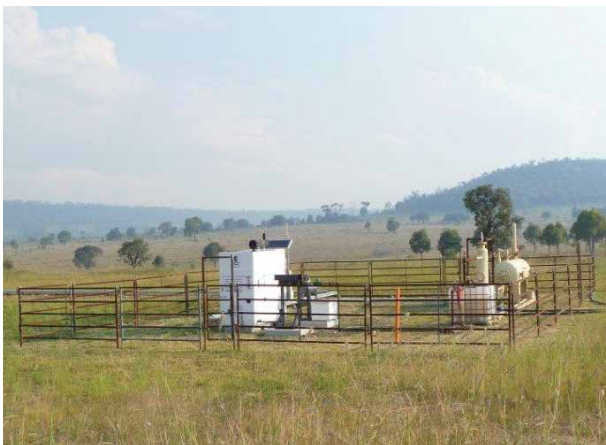
Well lease pad with cattle panels around the well lease surface infrastructure.
