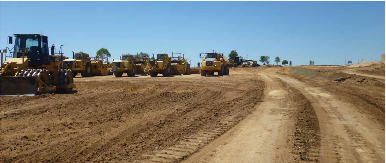
Machinery used during construction of a WMP.
