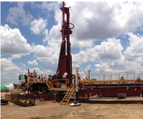
Installing conductor casing.
