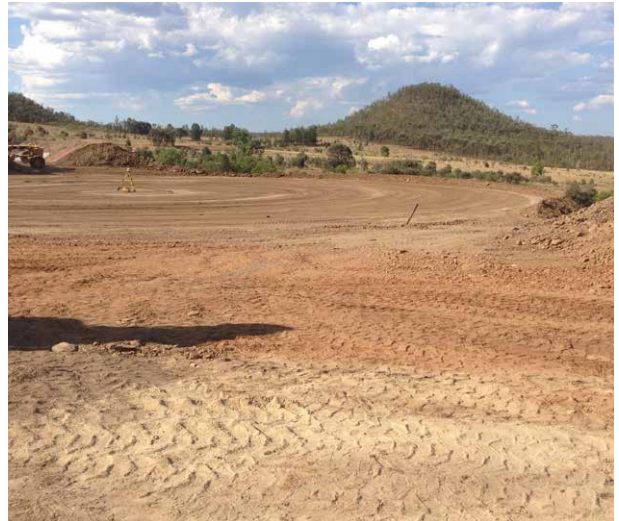
Construction civil works for a 3.6 megalitre MOWST.
