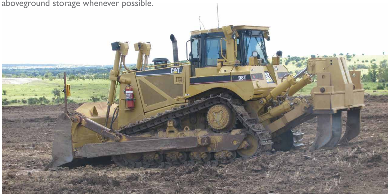
Example of a bulldozer on site.
