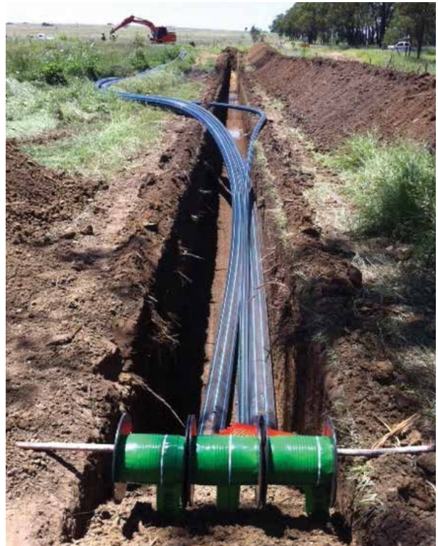
Three water flowlines in one trench.
