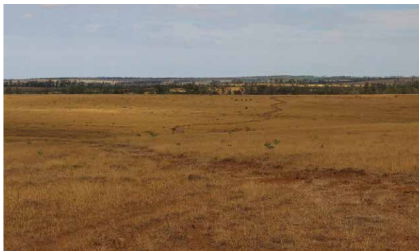
Example of a prepared seismic line through blade plough country. Seismic line has weaved around natural features to reduce clearing.
