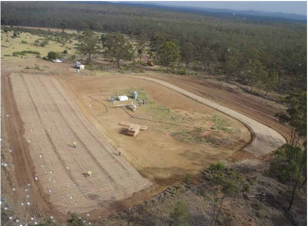
Stage 2 works execution complete.
