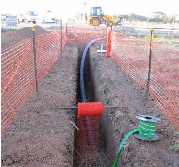
Single water flowline in trench.
