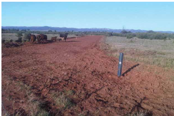
Reinstated flowline post-construction. The reinstatement is not yet complete.
