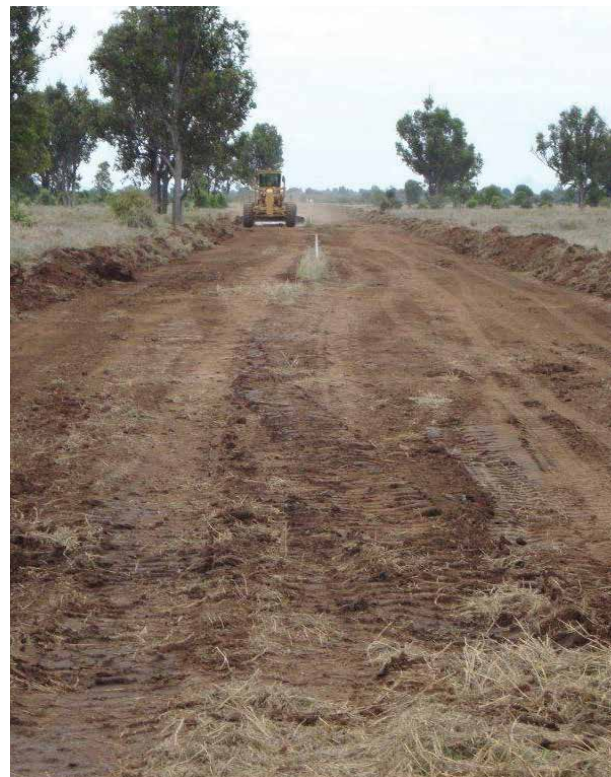
Clear and grade in preparation for flowline construction.
