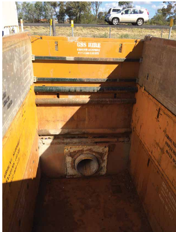
Example of a pipeline road crossing under a highway.
