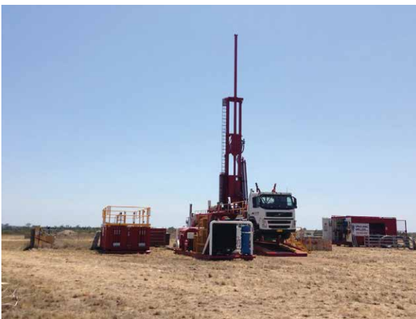
Rig with mud tanks and pumps.
