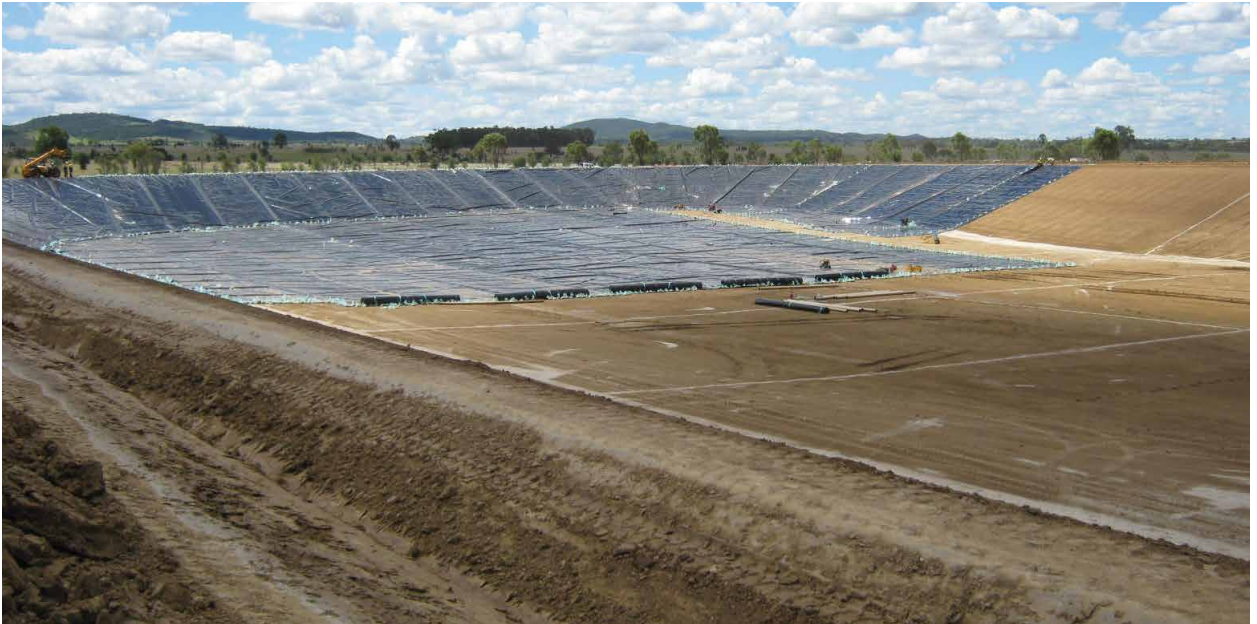
A HDPE membrane lining being laid into a WMP.
