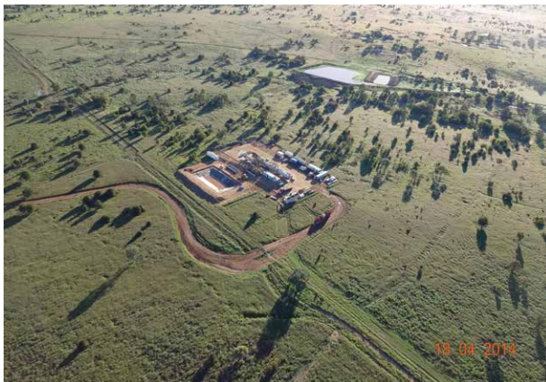
Minimal disturbance lease with a mud pit for the workover rig.
