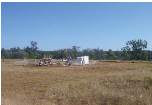
Well lease pad with grass cover returned and cattle panels around well lease surface infrastructure.
