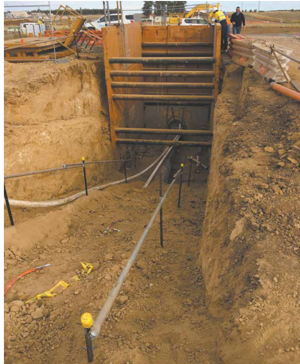
Example of a pipeline road crossing under a highway.
