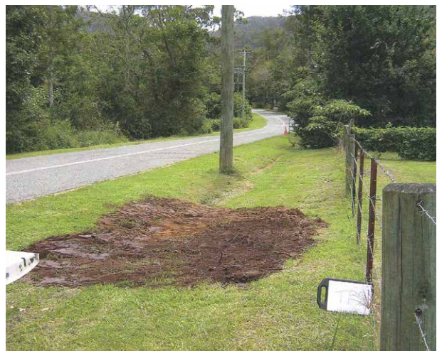
Backfill of test pit.
