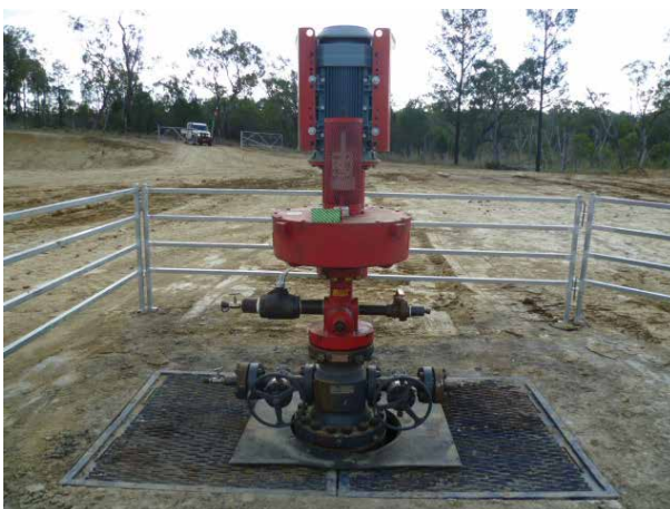
Completed wellhead with a pump installed.
