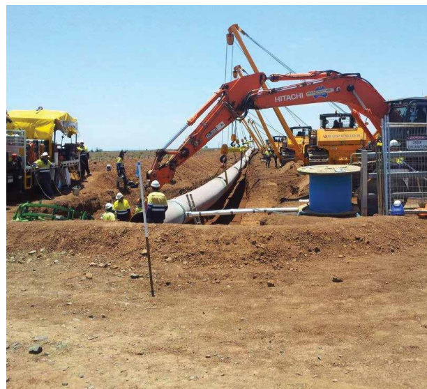
Pipe being laid into the trench.
