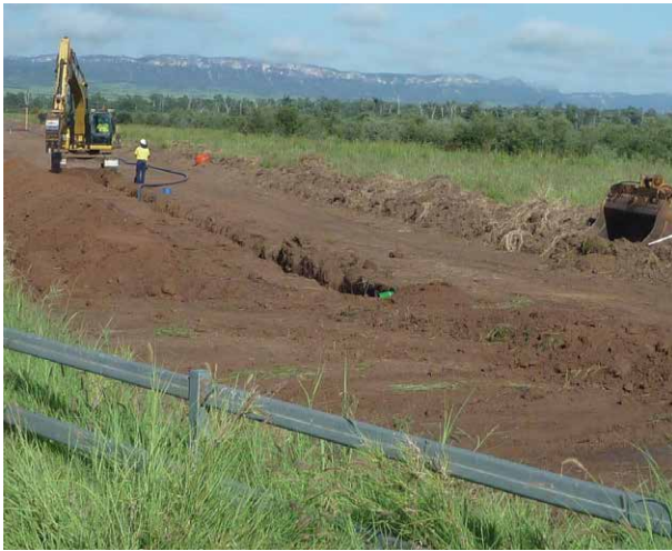
Flowline trenching and laying.
