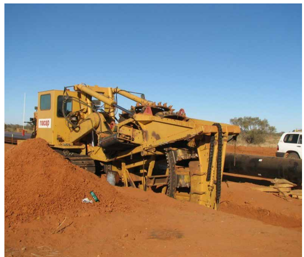
A bucket-wheel trenching machine..
