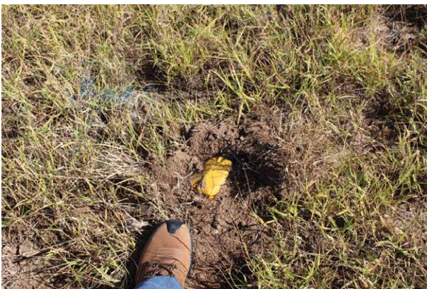
Wireless geophone installed in the ground, only the battery pack is visible.
