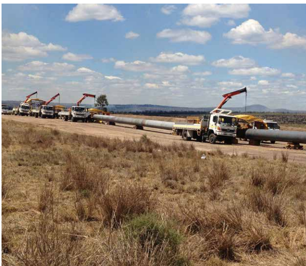
Pipe delivered to site and strung along the pipeline ROW.
