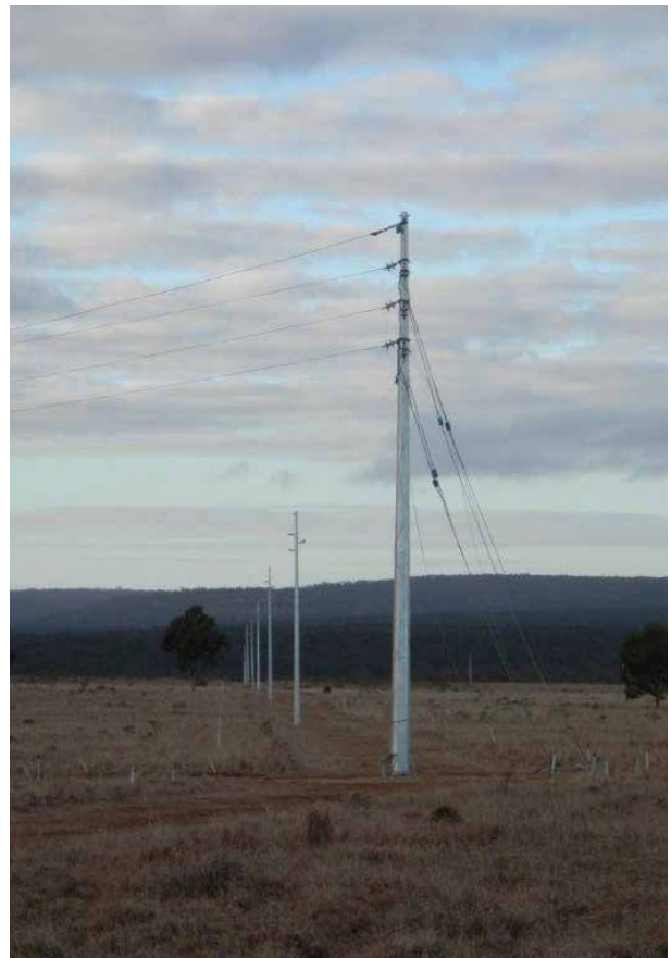
Completed aboveground powerline.
