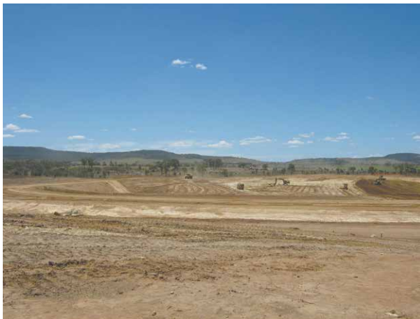
WMP under construction.
