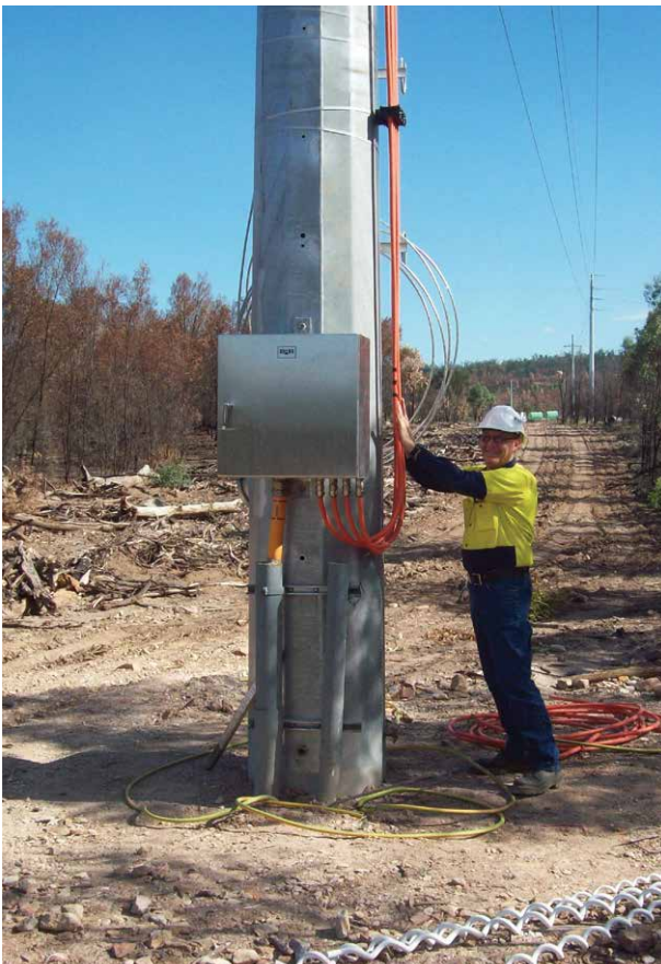
Aboveground powerline construction.
