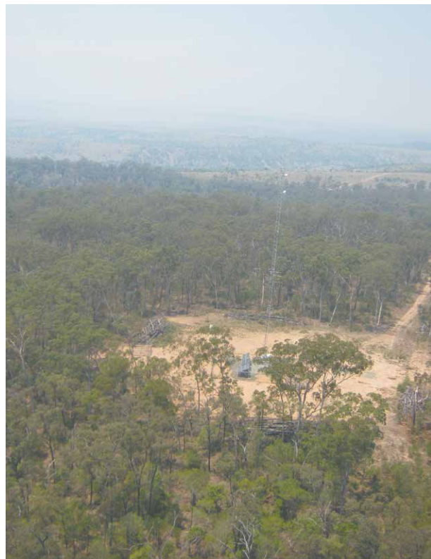
60 metre high communications tower.
