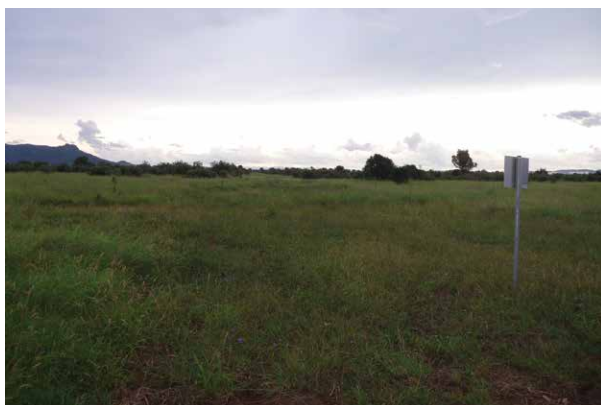
Example of a flowline 83 days after reinstatement when the reinstatement is complete.
