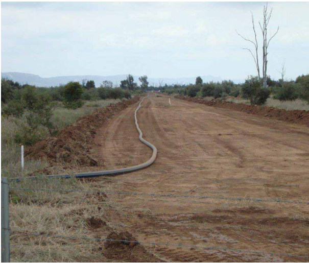
Water flowline stringing and welding once complete.
