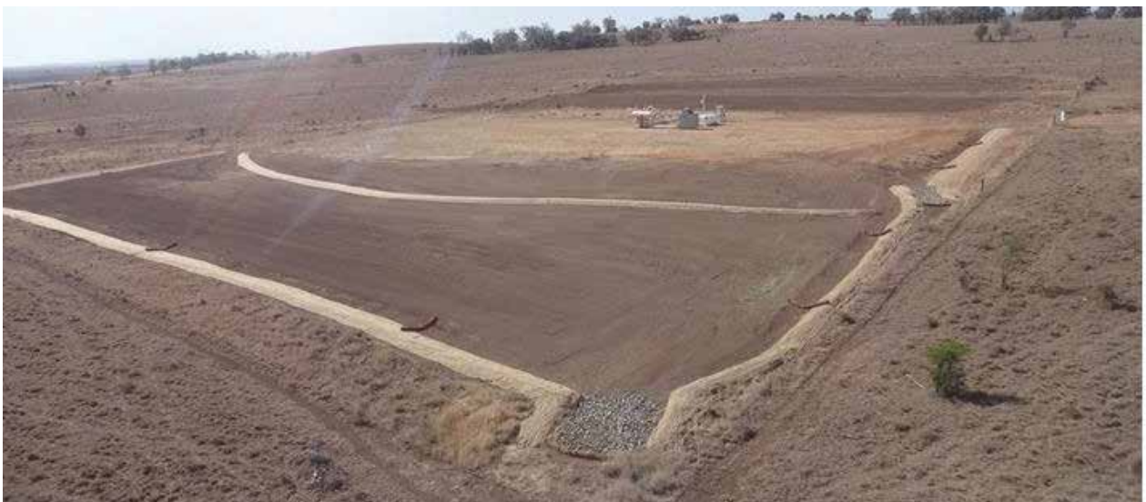
Stage 2 works execution complete.
