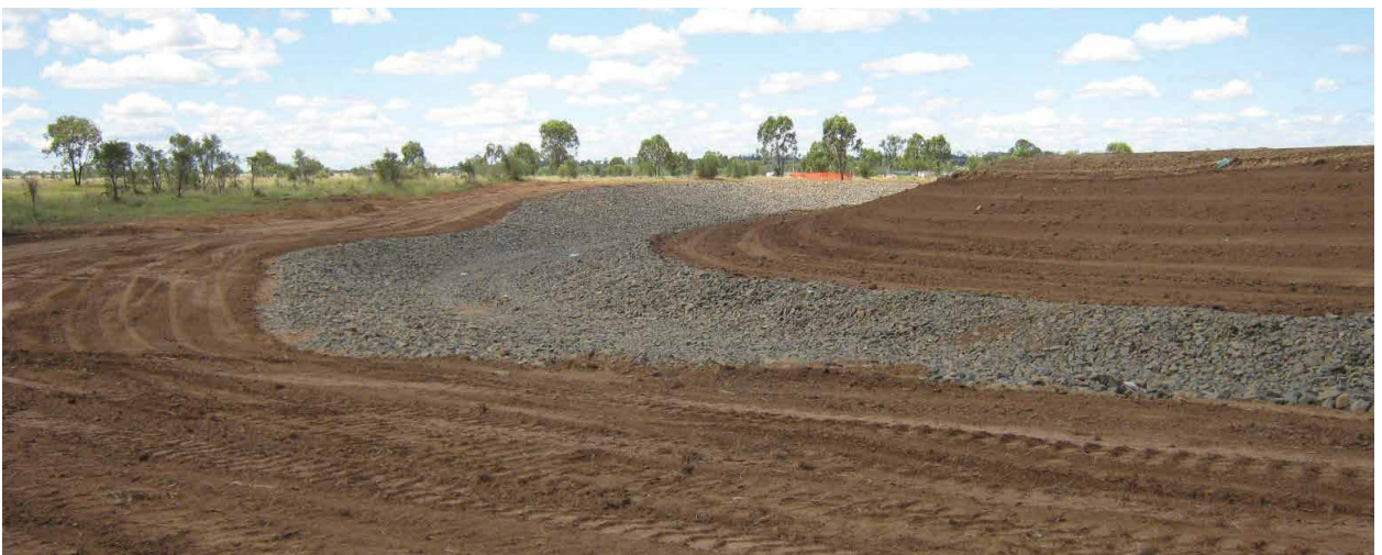
Spillway around the outside of the WMP walls.
