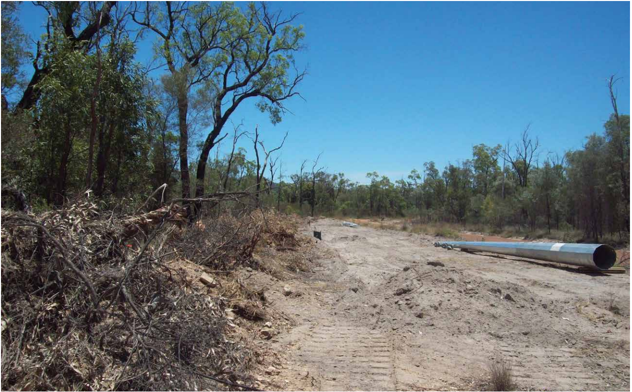
Aboveground powerline pre-construction.
