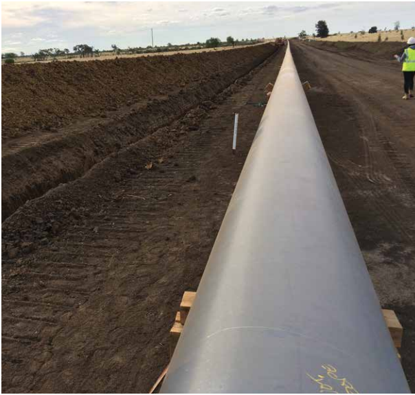
Trenching complete, ready for pipe to be laid.
