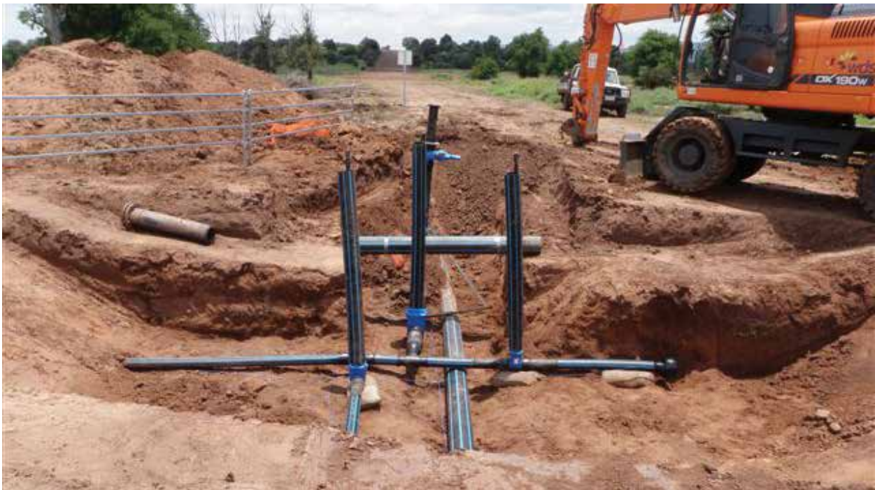
Construction of an underground HDPE manifold.
