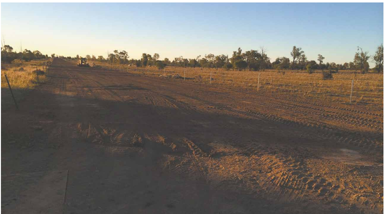
Example of a ROW after pipe has been buried.
