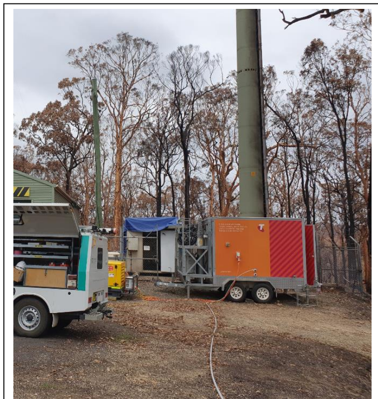
Figure 4: Cell on Wheels with fire damaged mobile network facility in the background (blue tarpaulin covering), Malua Bay NSW
