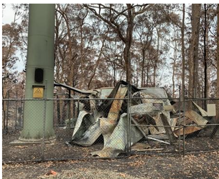
Figure 3: Fire-damaged mobile network facility, Surf Beach NSW
