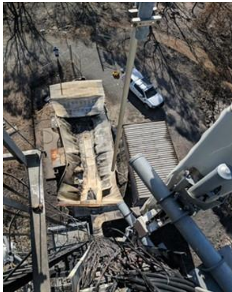
Figure 2: Fire-damaged mobile network facility, Mount Torrens SA
