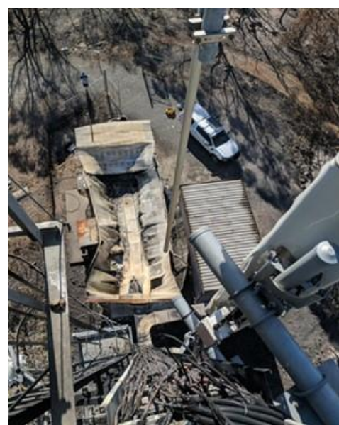
Figure 2: Fire-damaged mobile network facility, Mount Torrens SA
