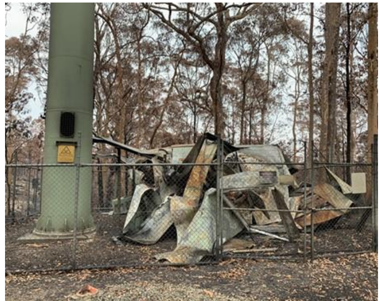
Figure 3: Fire-damaged mobile network facility, Surf Beach NSW
