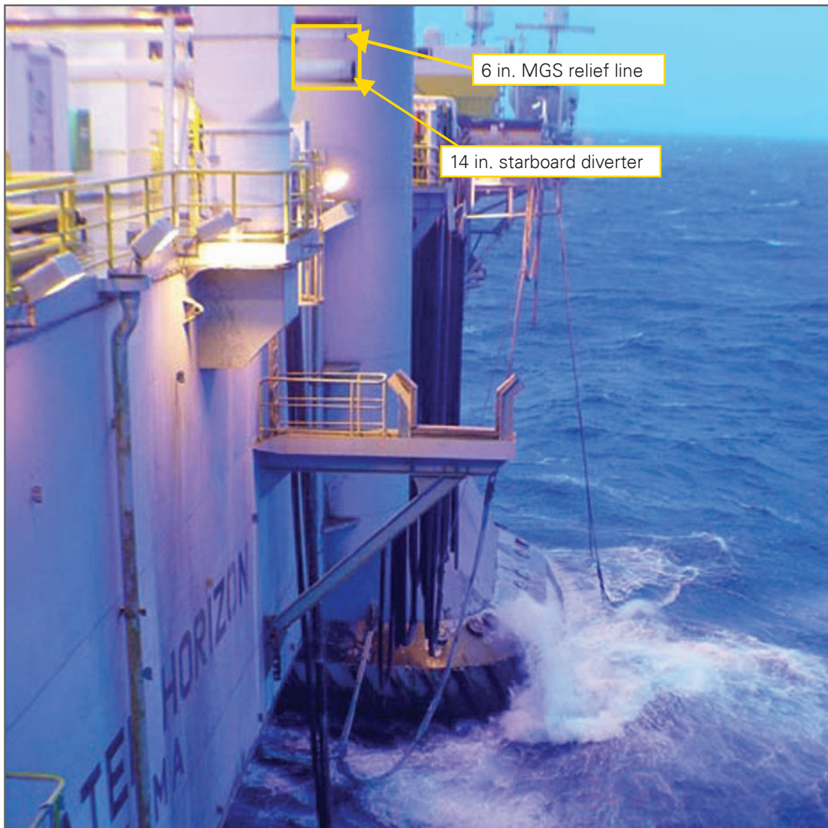
Figure 6. Photograph of Starboard Overboard Lines.
