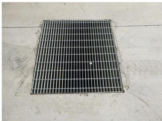
Both grates below were non-compliant and unidentifiable.
