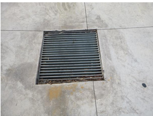
Both grates below were non-compliant and unidentifiable.
