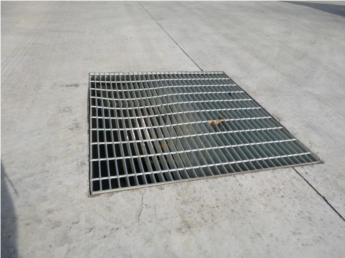
Both grates below were non-compliant and unidentifiable.
