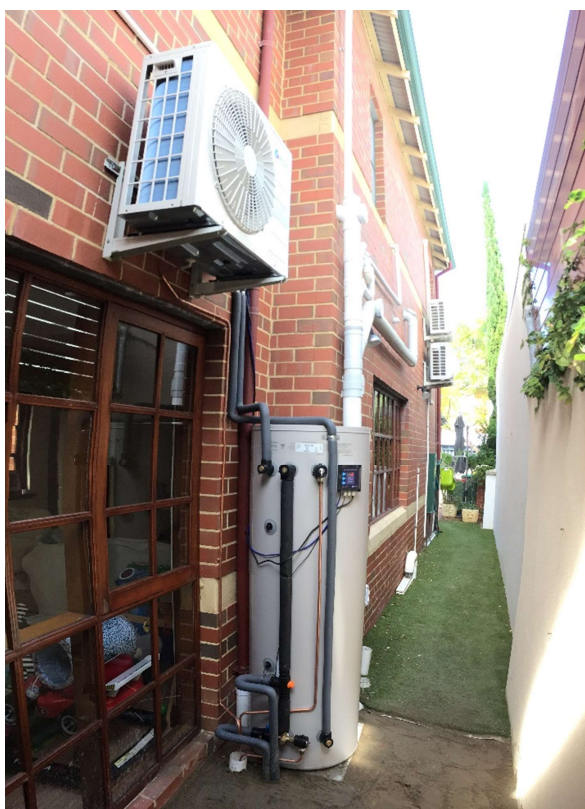
Figure 9 - Air Source Heat Pump for hot water
