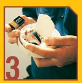
Change the battery at least once a year with the battery specified by the alarm manufacturer.
