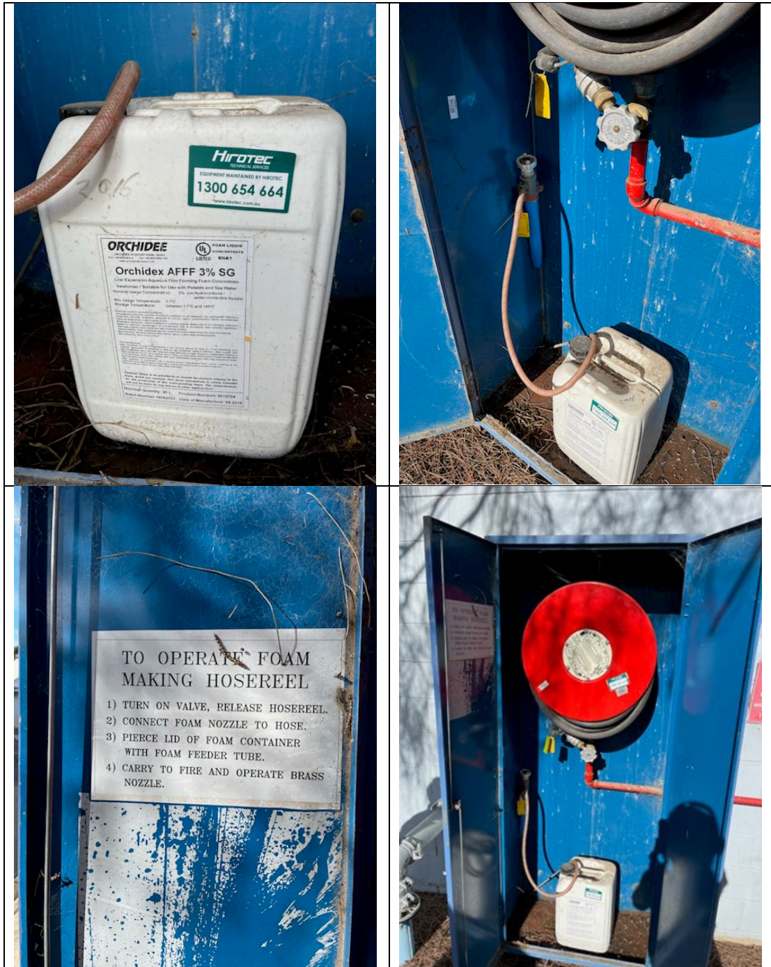
C6 PFAS foam-fed fire fighting installation within Airservices' Melbourne Airport compound
