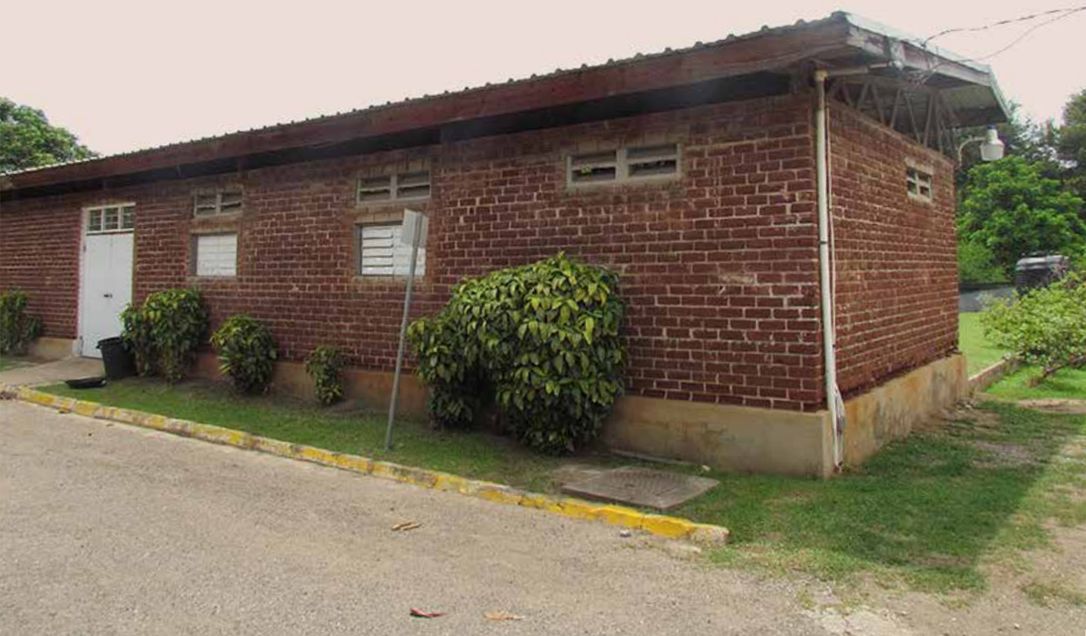
Construction using bricks made from residue
