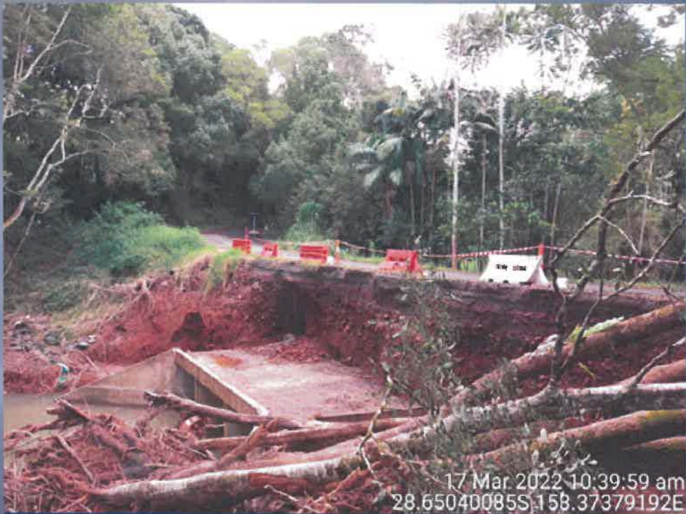
Dunoon Rd: Culvert washout
