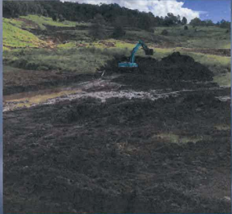
24t excavator clearing landslip over Bice Rd, Leycester
