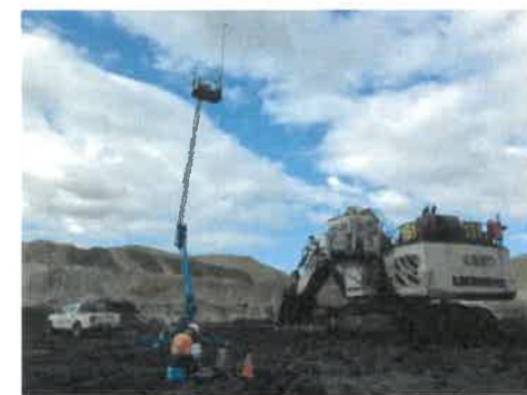
Sound Attenuated Machinery to reduce noise emissions from machinery
