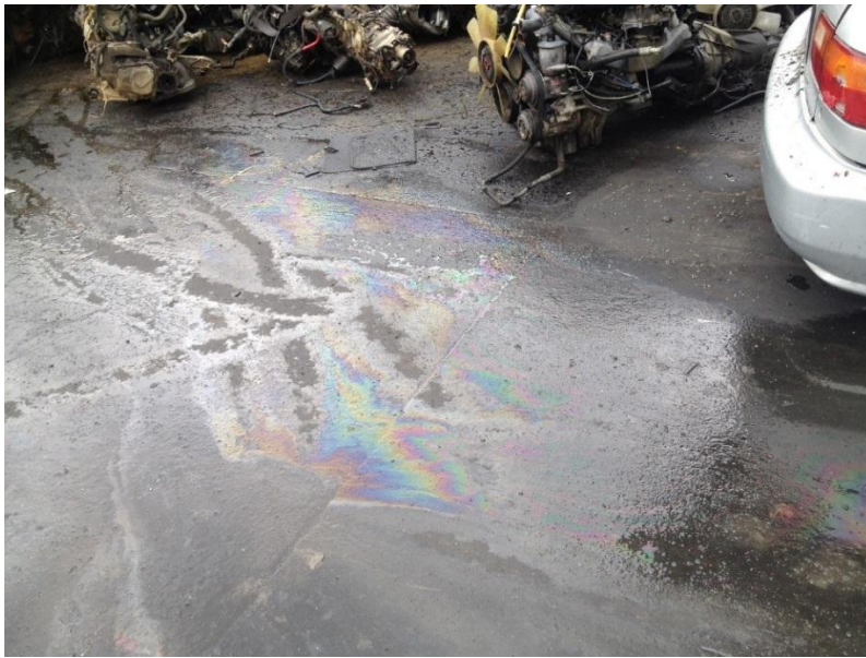
21.2 Figure 22: Substantially non-compliant worksite, oils and fuels on ground create a slip hazard
