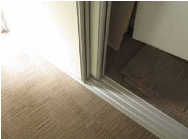
Flush BIR floor threshold, Mission Australia (Victoria) housing, MSM Architects
