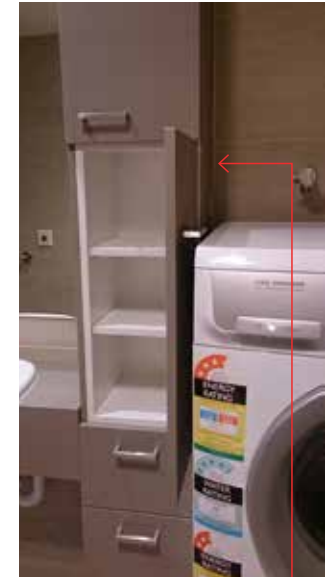
Bathroom vertical tower cabinet (left) with hole added for use of appliances at basin (right)
