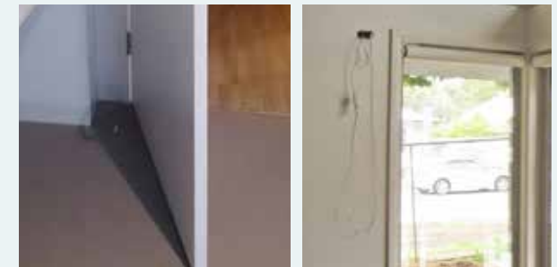
Slimline wall corner guards and timber-look vinyl flooring, Abbotsford (left) and pre-wiring for future blind automation prior to install of coverplates, TAC RIPL Housing (right).
