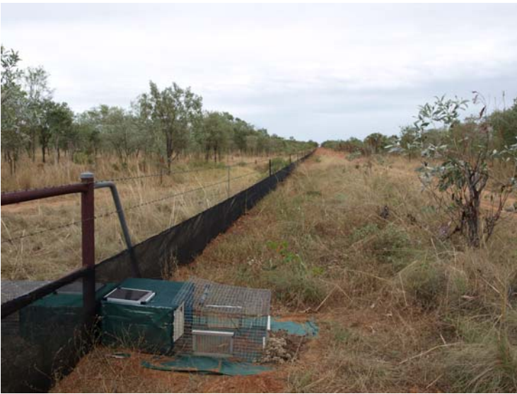
Figure 2. The barrier/deflection fence at Gregory's Tree. There is no evidence that the fence is providing any benefits. Photo: A. Peacock
