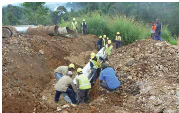
Komo station road being fixed. Photo credit: James McIlraith/University of Otago.
