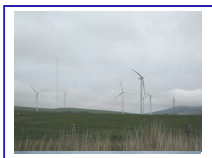
View of turbines at Waubra wind farm
