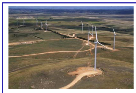
View of turbines at Capital wind farm
