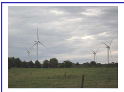
View of turbines at Wonthaggi wind farm
