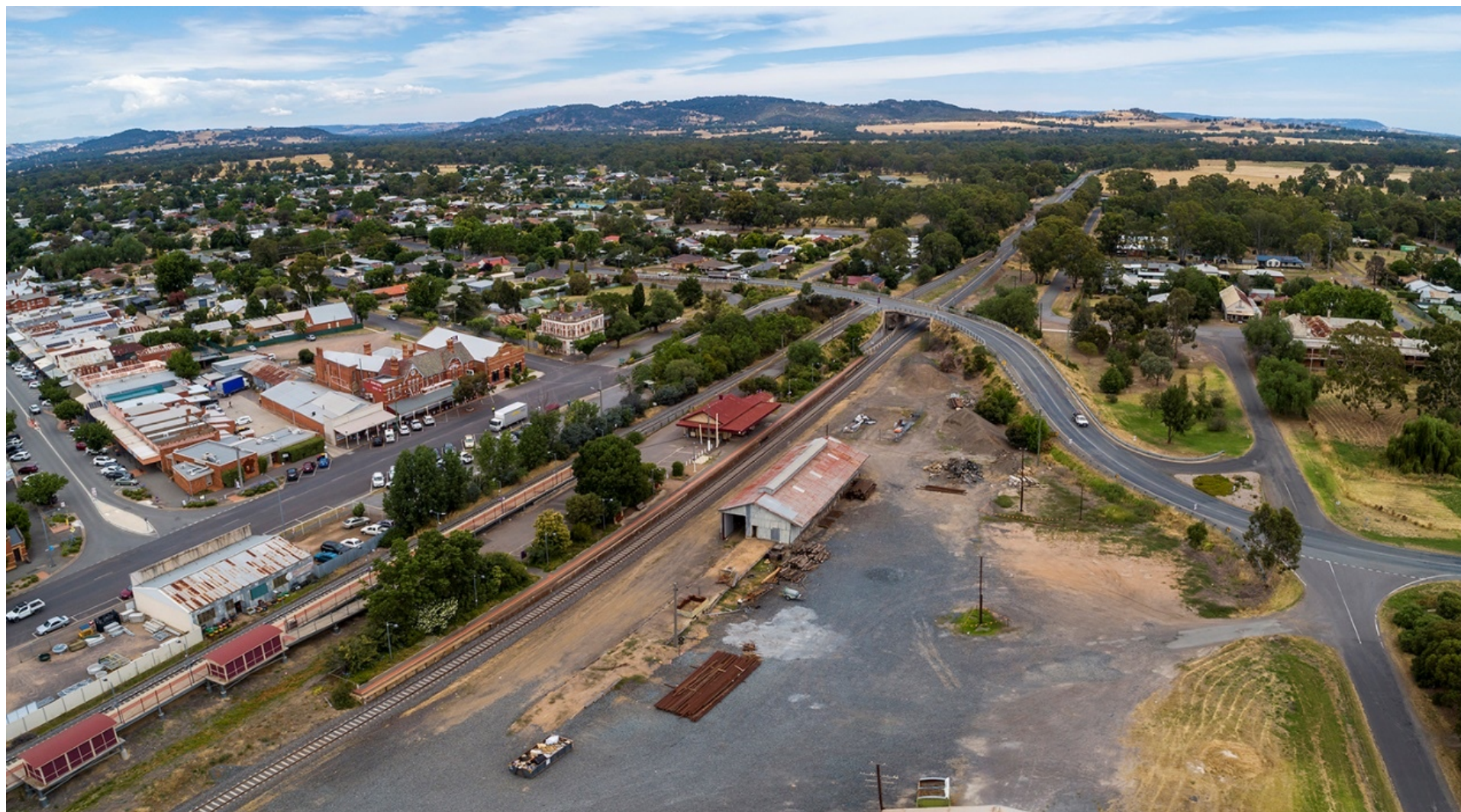
Existing rail crossing
