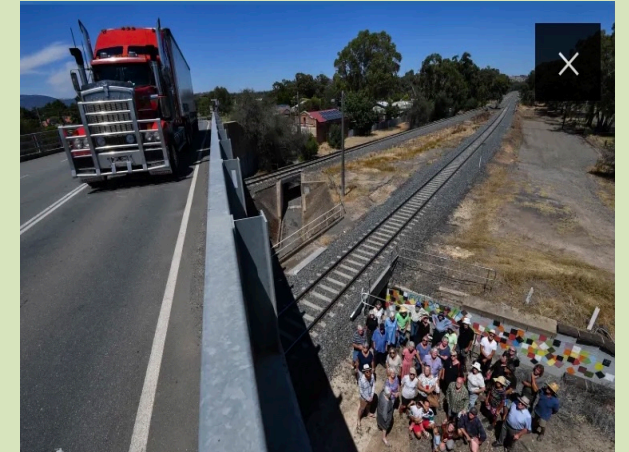
The road overpass between east and west Euroa. Source : Joe Armao, 'the Age' newspaper
