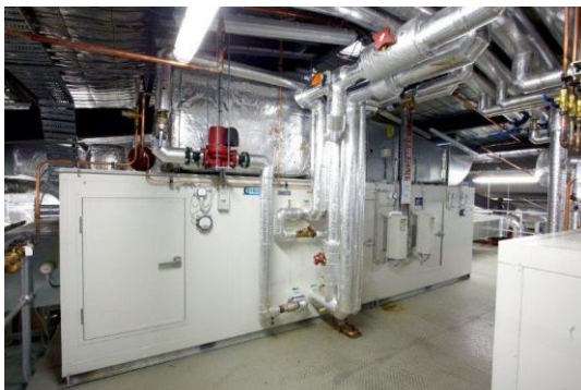
1. Specialised air handling systems ensure sterile air is passed into the compounding facility
