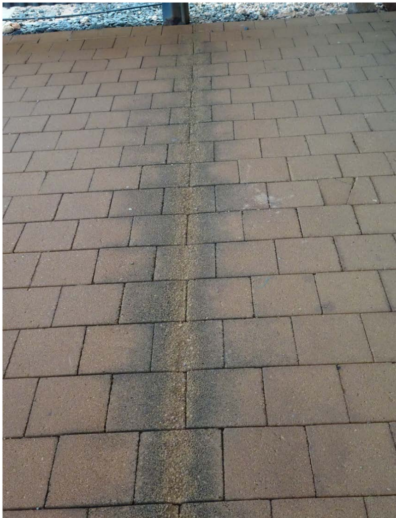
Figure 2: Effect on brickwork of 'acid rain' from gap in roofing at Woodside Visitor Centre, July 2016
