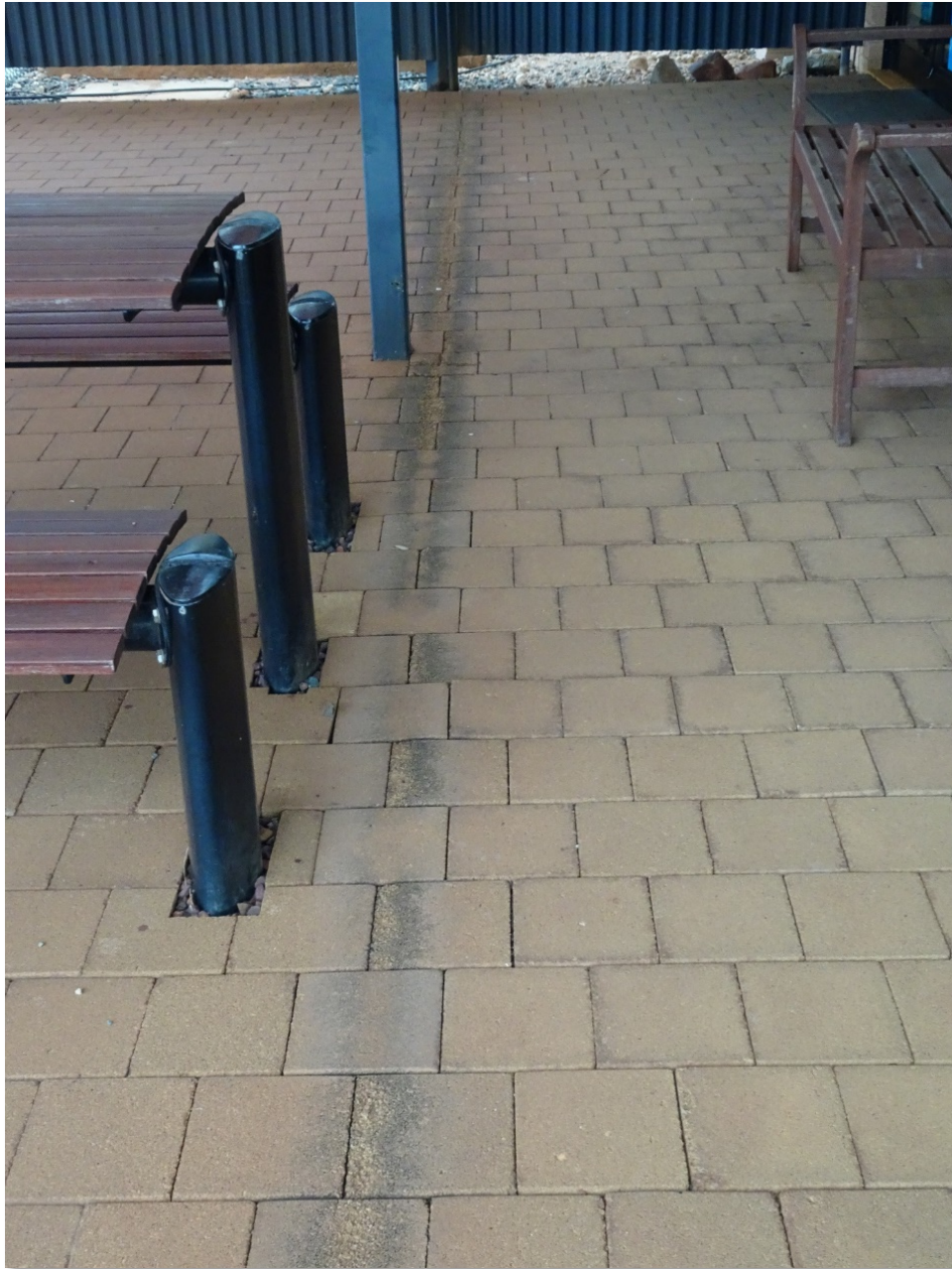
Figure 3: Effect on brickwork of 'acid rain' from gap in roofing at Woodside Visitor Centre, July 2016
