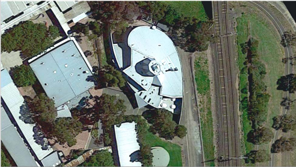
VSSEC occupies a purpose-built facility at Strathmore Secondary College in Melbourne. The building's shape represents the arms of a spiral galaxy.
