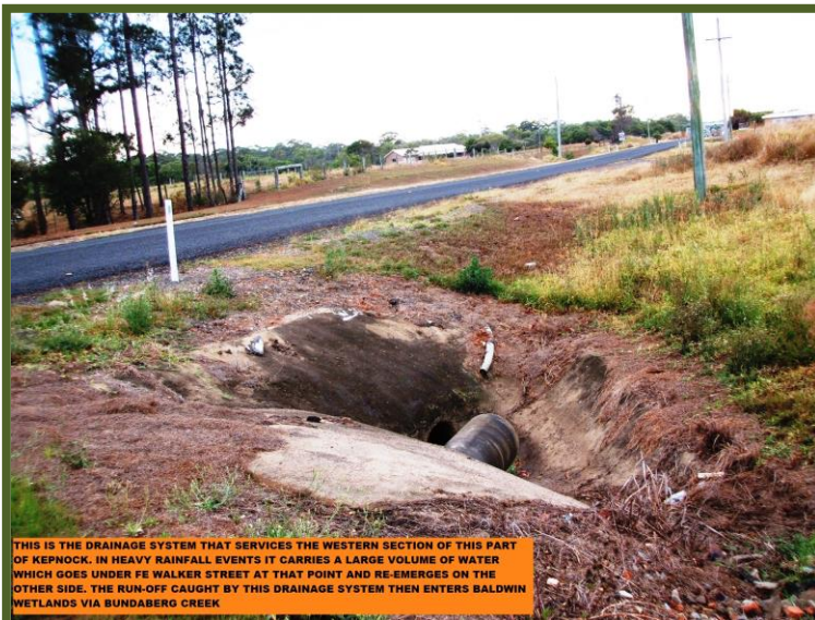
CULVERT E – drains the homes to the north-west
