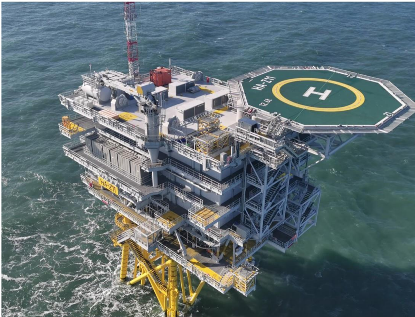
One of the fixed offshore substations used at the Hornsea One project. Image courtesy of Orsted. All rights reserved.
