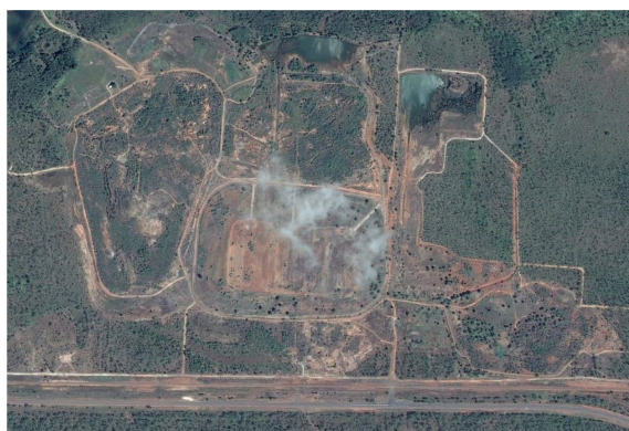
Figure 9: Aerial views of the former Woodcutters Pb–Zn–Ag mine, NT—(top) prior to rehabilitation in 1998 (Taylor & Pape, 2007); (bottom) recent site view 17 May 2016 (GE, 2016) (note: north is pointing to the right)
