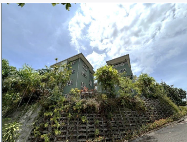
Retaining wall showing typical topography.
