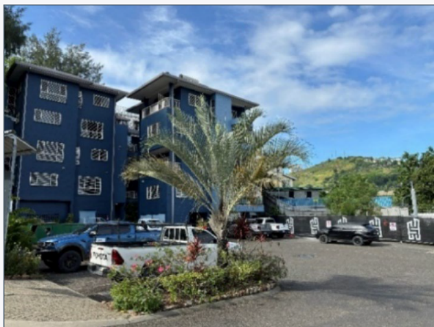
The base of the compound is relatively flat but the majority of residences are built on a steep hill.
