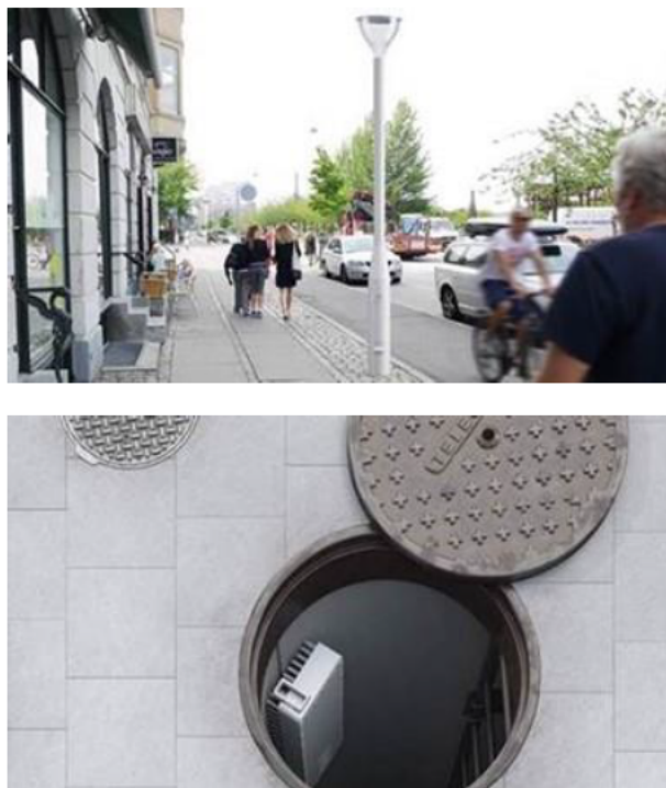
Figure 7: Future 5G small cell deployments, Top – antenna on street light pole; Bottom – base station equipment in access hole Courtesy, Ericsson
