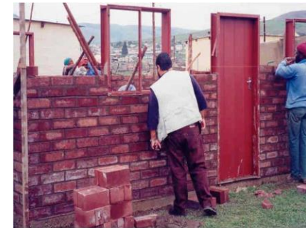
Affordable housing under construction using Nu-Rock Blocks in South Africa.
