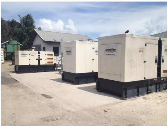
Image 2: Potable Water Production Upgrades – Water Production Generators – Nauru Utilities Corporation
