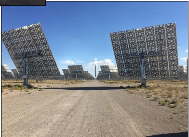
Looking back to the solar tower at the centre of the field through the array of heliostats. Each heliostat is made up of 35x1.8 m mirror facets, yielding a heliostat overall usable area of 115.7 m<sup>2</sup>. Total solar field aperture adds up to 1,196,778 m<sup>2</sup>.
