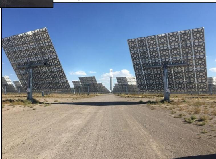
Looking back to the solar tower at the centre of the field through the array of heliostats. Each heliostat is made up of 35x1.8 m mirror facets, yielding a heliostat overall usable area of 115.7 m<sup>2</sup>. Total solar field aperture adds up to 1,196,778 m<sup>2</sup>.
