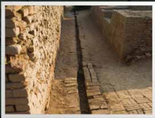
1. MOHENJO-DARO, DRAINAGE SYSTEM
