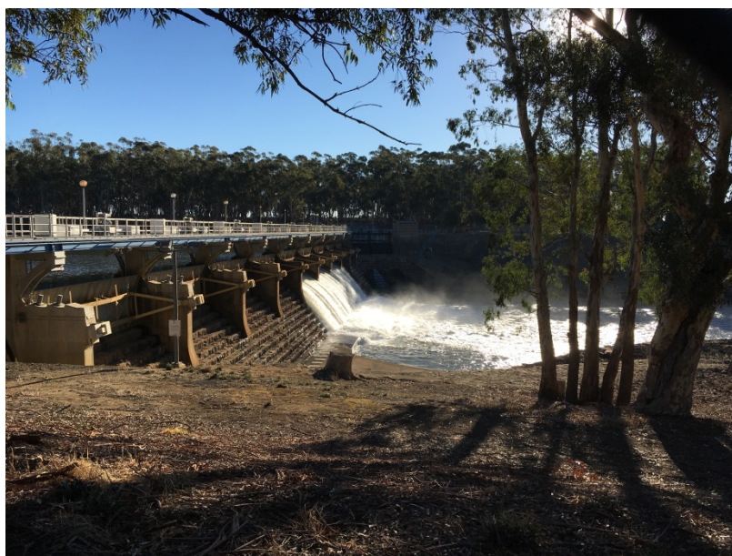
Goulburn River weir
