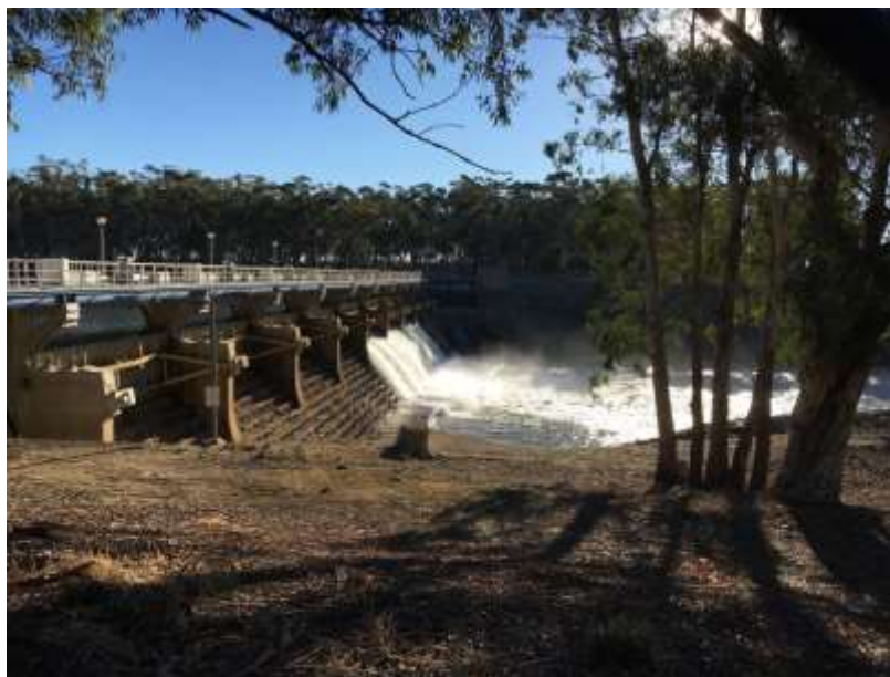
Goulburn River weir
