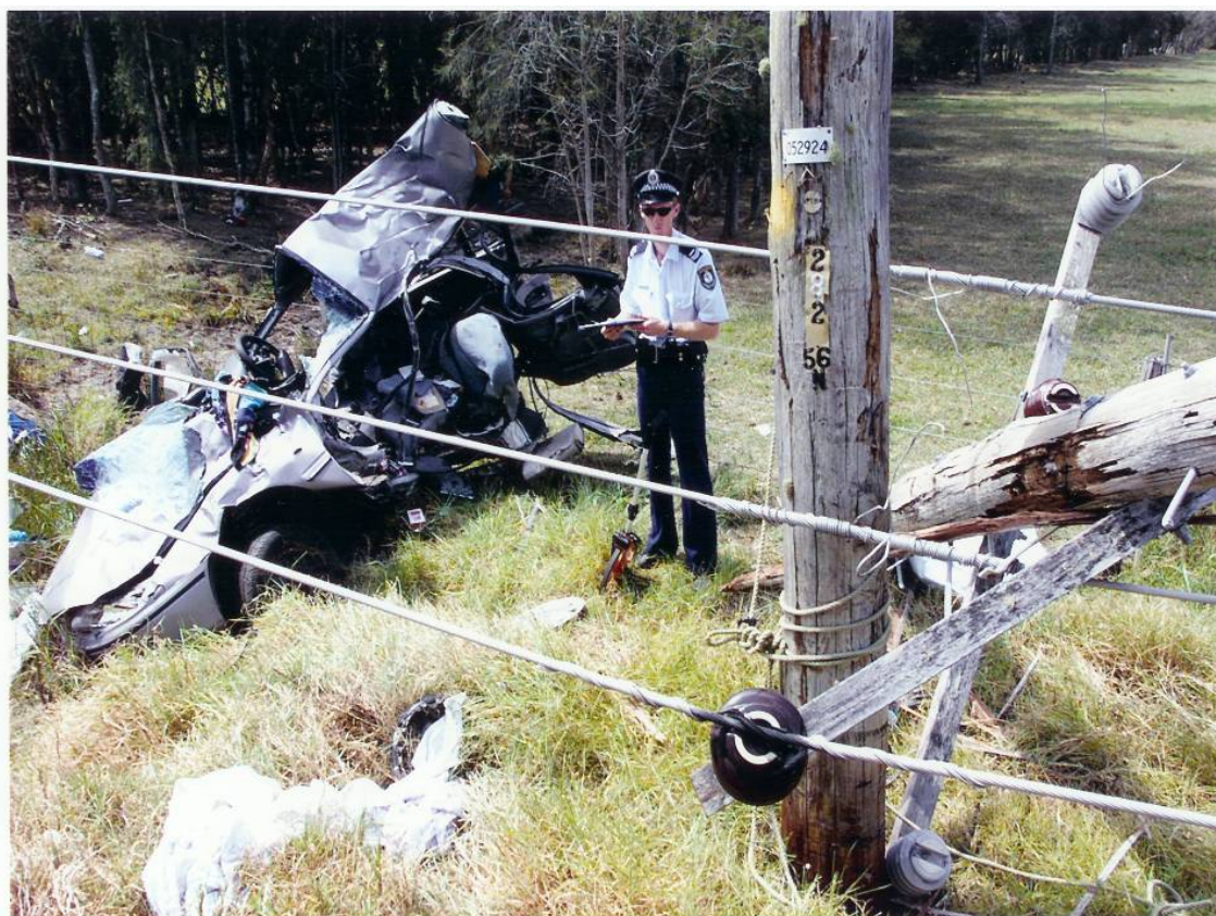
Figure 4: Electricity pole destroyed and lines brought down by an errant road vehicle; imagine the impact on life-line telecommunications if the government-mandated National Broadband Network had been attached to this pole!
