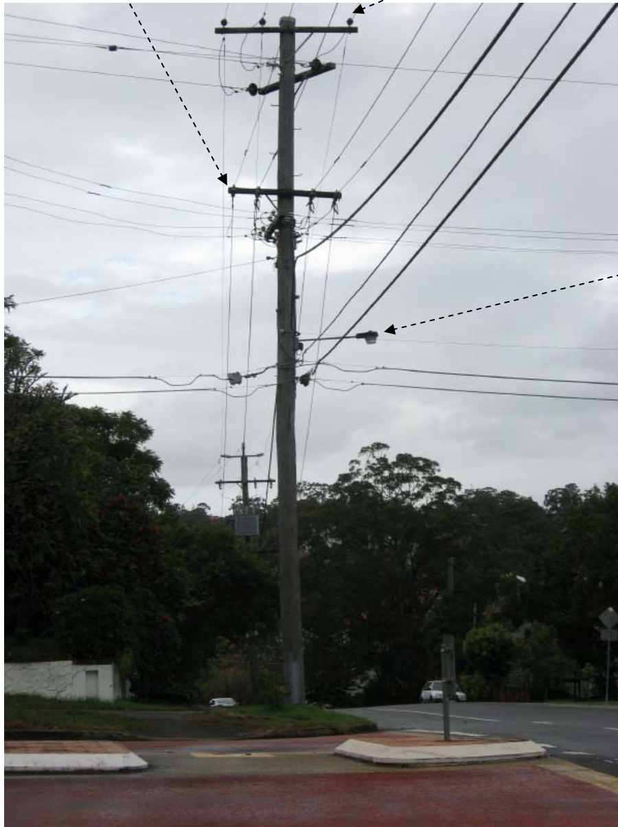
Figure 2: A pole at the corner of Abbotsleigh Street and Geelong Avenue (suburb of Holland Park, Brisbane) adjacent to that of Figure 1 - illustrating the added complexity of lines and cables arising at a typical street intersection, together with the higher potential for being struck by road vehicles.
