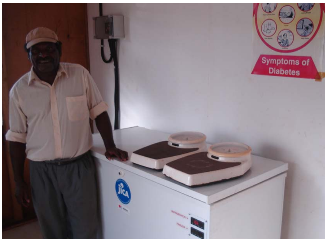
Solar fridge installed at Buzi
