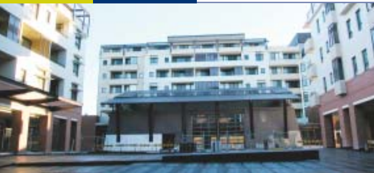
Kogarah Town Square – energy efficient design and roof-integrated PV
