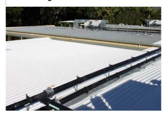
The temperature on the near roof painted with heat-reflective paint is 18° cooler than the far roof yet to be painted.
