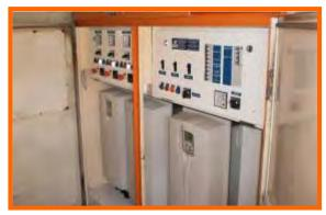
New switchboard with variable speed pump drives
