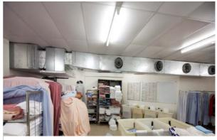
Chilled water is used to air-condition the home's large laundry, saving a significant amount of energy over conventional DX air-conditioning.
