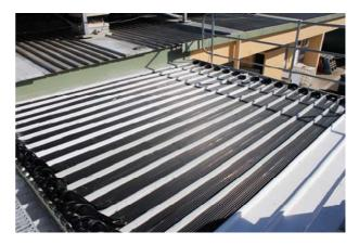
The DIY solar water heater uses pool blankets coiled on the rooftop.
