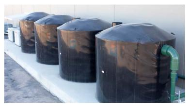
The thermal energy storage tanks effectively operate as a battery in the system, allowing the building cooling system to be decoupled from the process plant.
