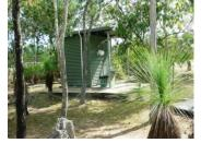
The metal construction of the Coen model which cost in the order of \$12,000 installed is more likely to survive the ravages of bush fire and termites.
