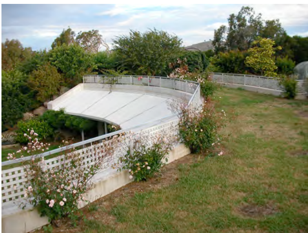
Earth covered house built into the hill at Tooborac in 1985 not only for aesthetic reasons but for the practical consideration that it was in a bush fire prone area.
