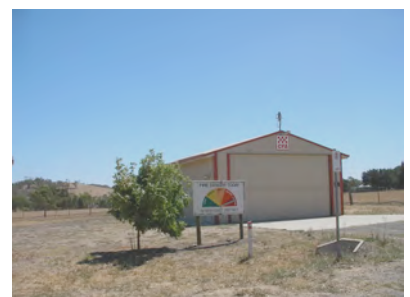
Tooborac Fire Station
